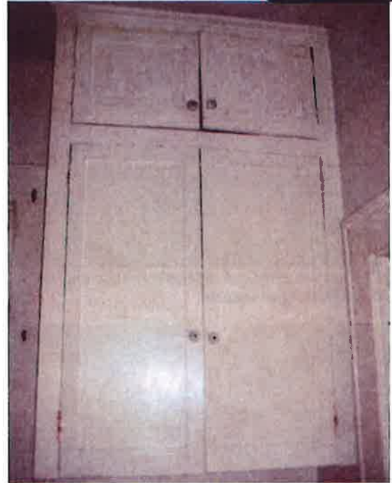
2 - Original Upper Cabinet in Kitchen
