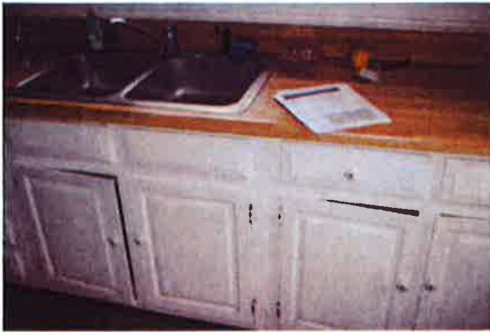
5 - Kitchen Cabinets (lower) - to be replaced matching existing original
