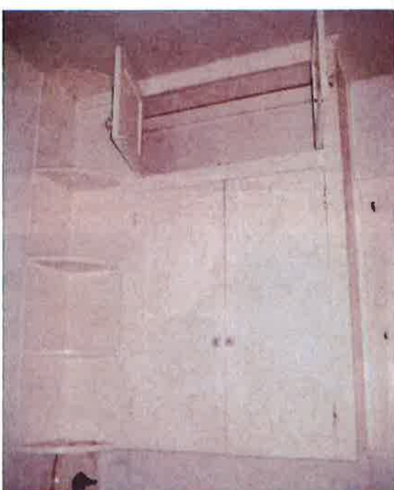
4 - Original Upper Kitchen Cabinet
