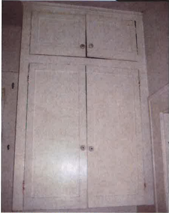
2 - Original Upper Cabinet in Kitchen
