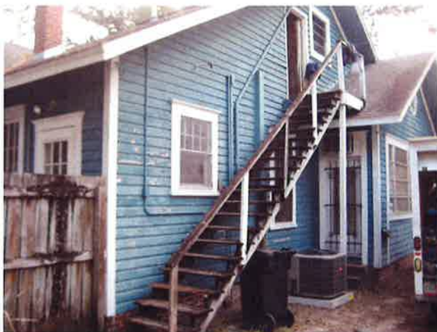
15 - Exterior Stairs to Attic - to be removed
