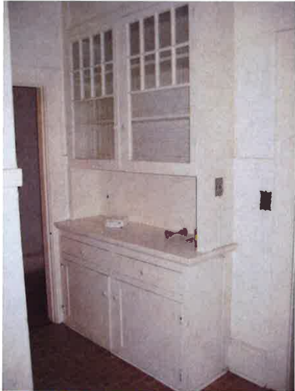
1 - Original Built-In in Kitchen
