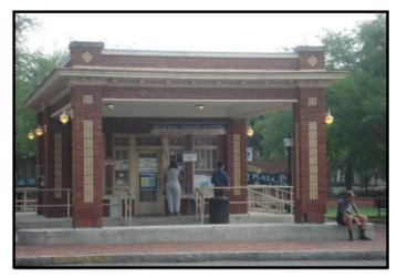
Despite its small size, the building boasts four doors, four full size windows and two smaller windows adjacent to the main door. The exterior brick is in generally good condition. However, other exterior features, such as the flat roof and woodwork around doors and windows, will require repairs.
