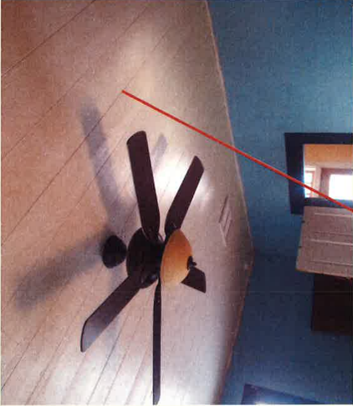
Uncovered and repaired old wood ceiling in master bedroom
