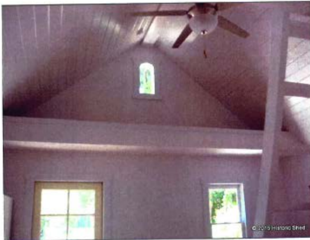
A 2' deep storage shelf was installed opposite the loft
