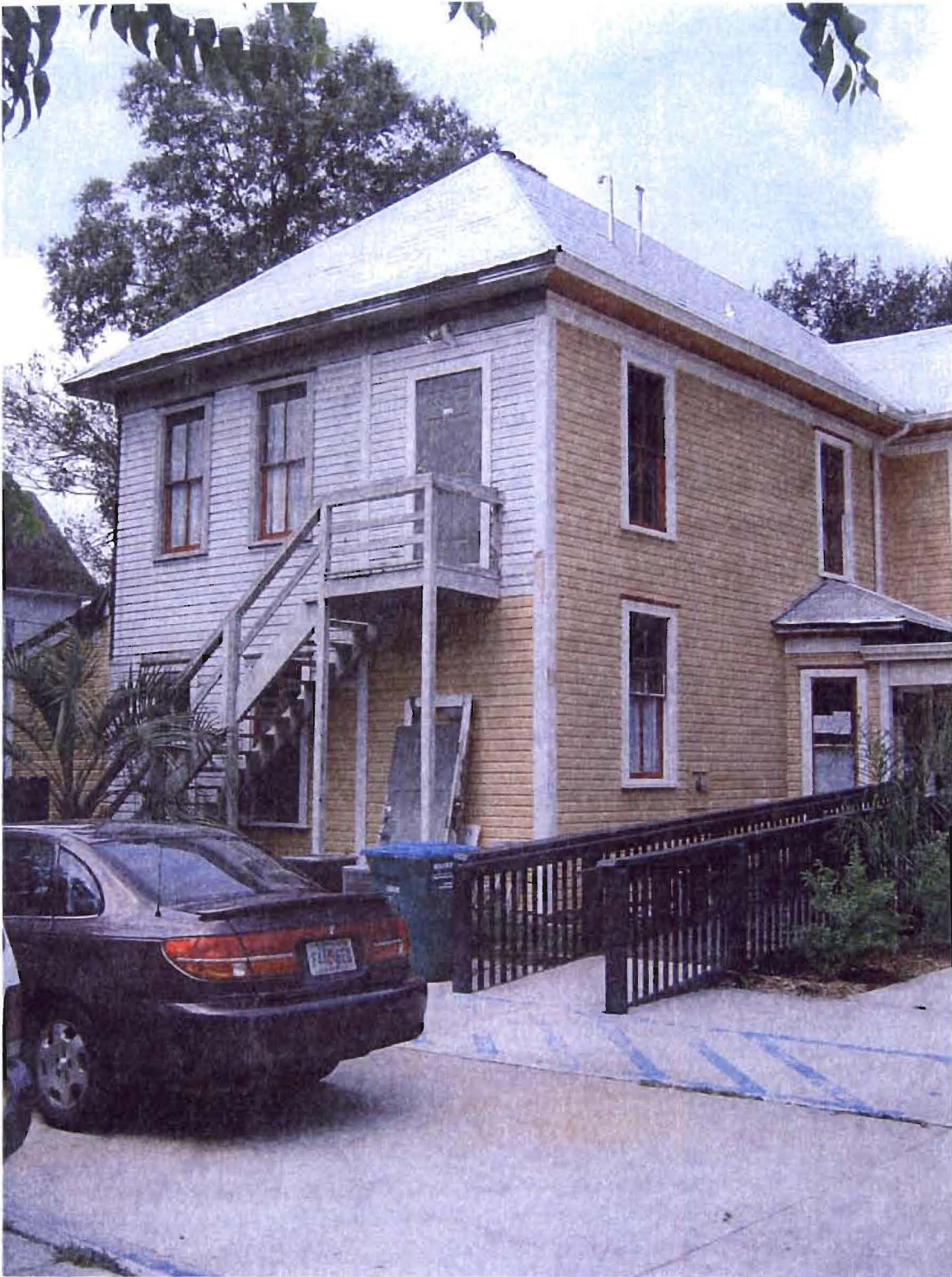
Looking SW from the existing parking lot.
