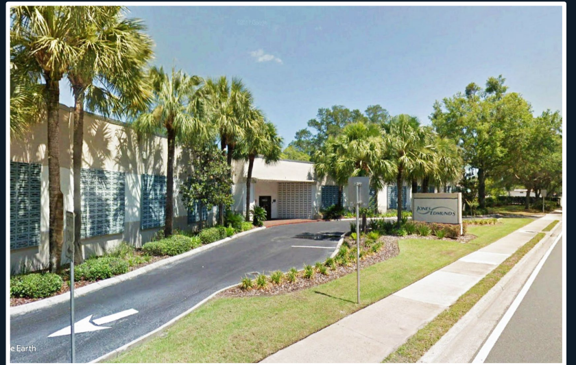
Existing Building on Private Property
