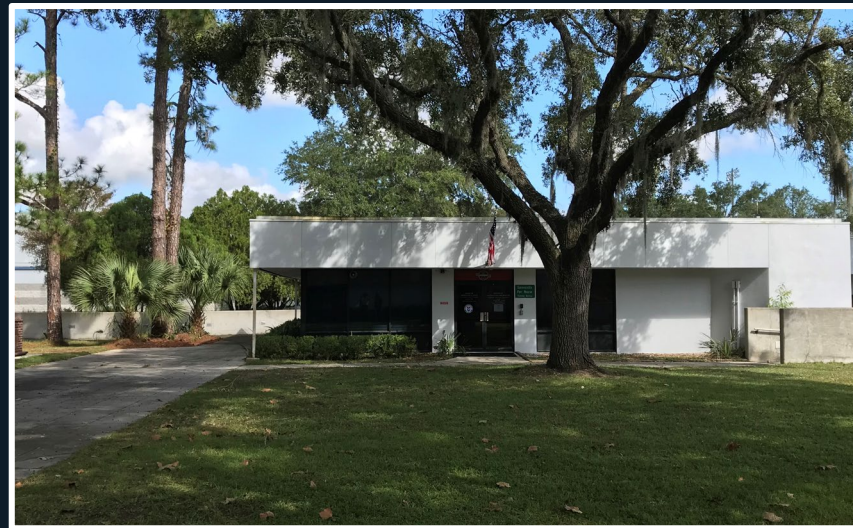
Gainesville Fire Rescue Admin. Building
