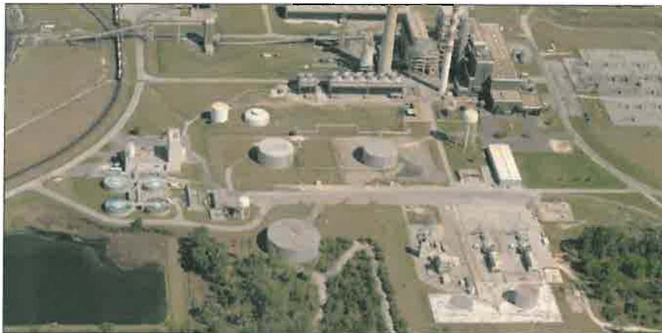
MAIN PLANT LOOKING EAST
