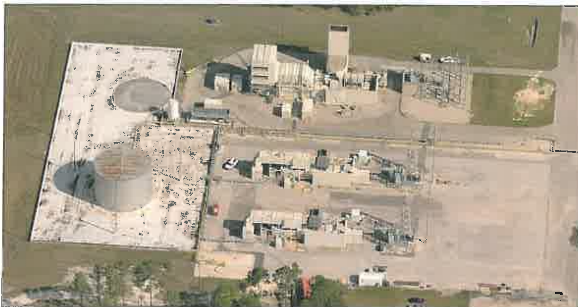
COMBUSTION TURBINES GT01, GT02 AND GT03
