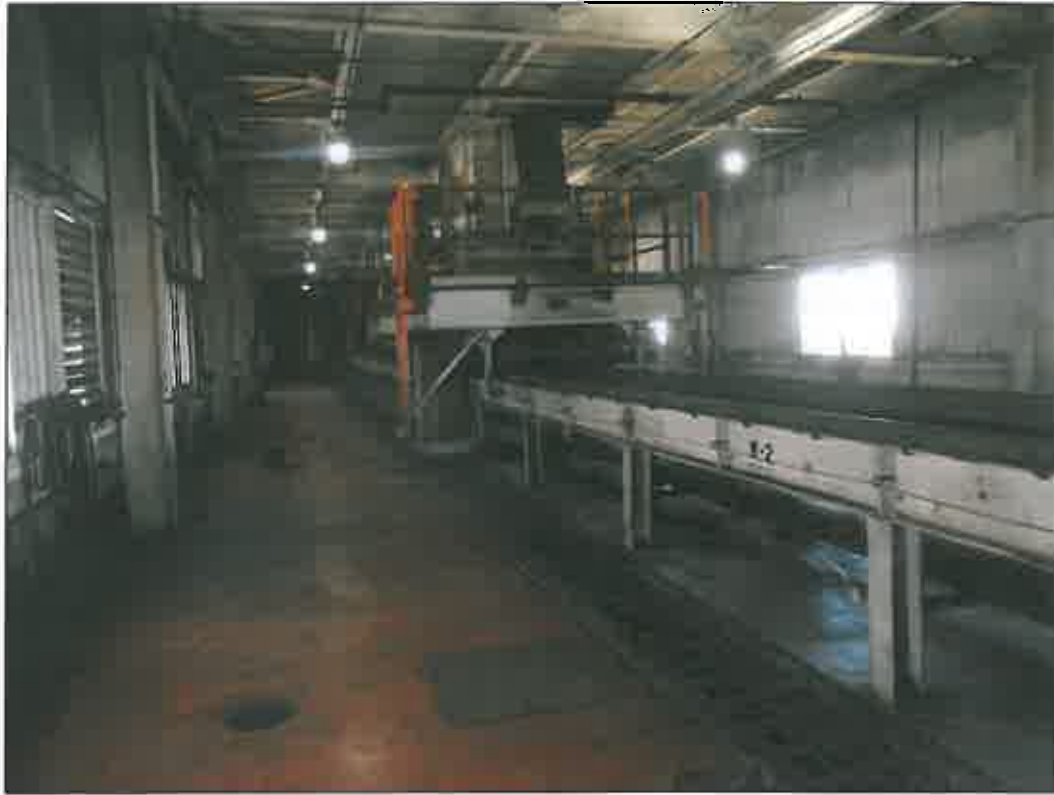
UNIT 2 TRIPPER FLOOR AREA
