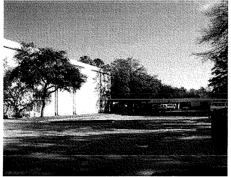
View of the West Side of the Center and Parking lot where the building expansion would take place.
