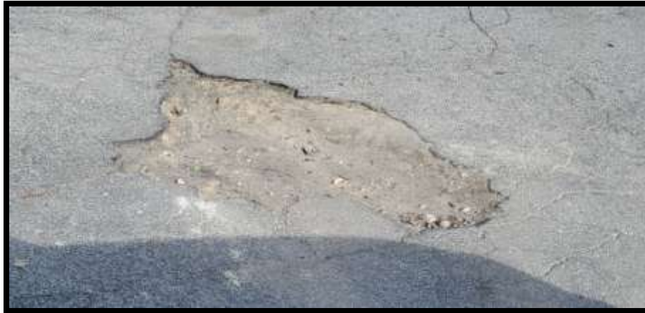
Potholes in Parking Lot #10, the appraiser counted at least a dozen similar potholes and asphalt damage
