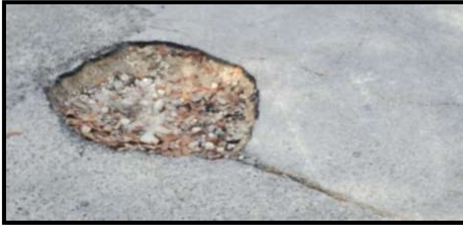
Potholes in Parking Lot #10, the appraiser counted at least a dozen similar potholes and asphalt damage
