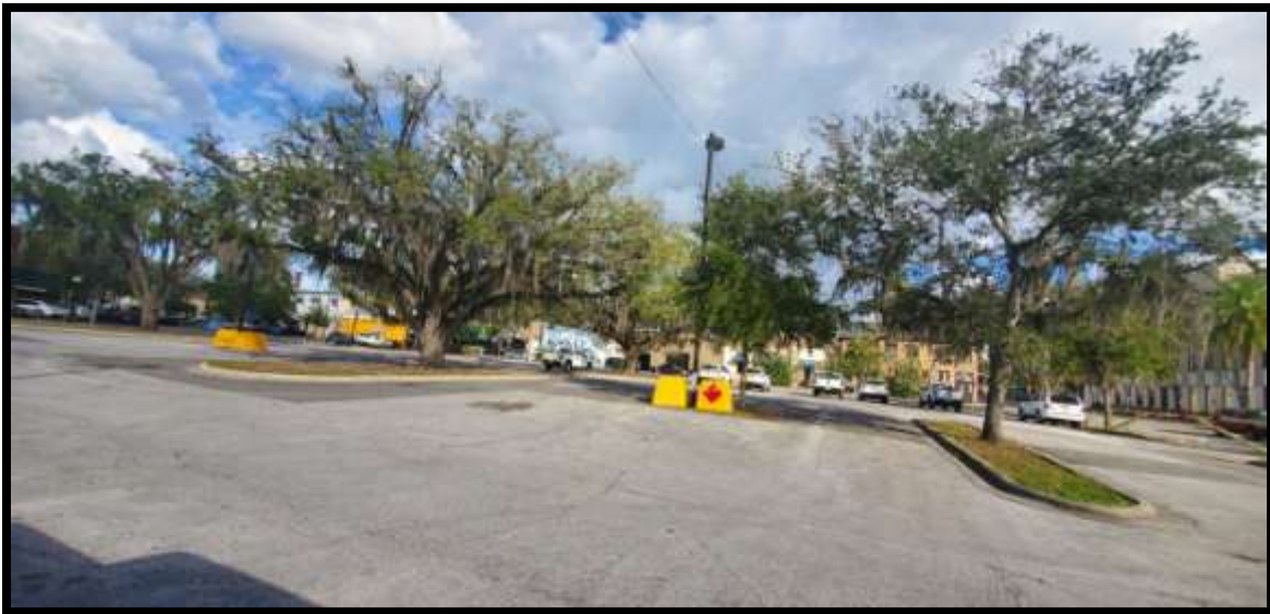
Interior parking lot view of trees, lighting, concrete blocks to protect light poles
