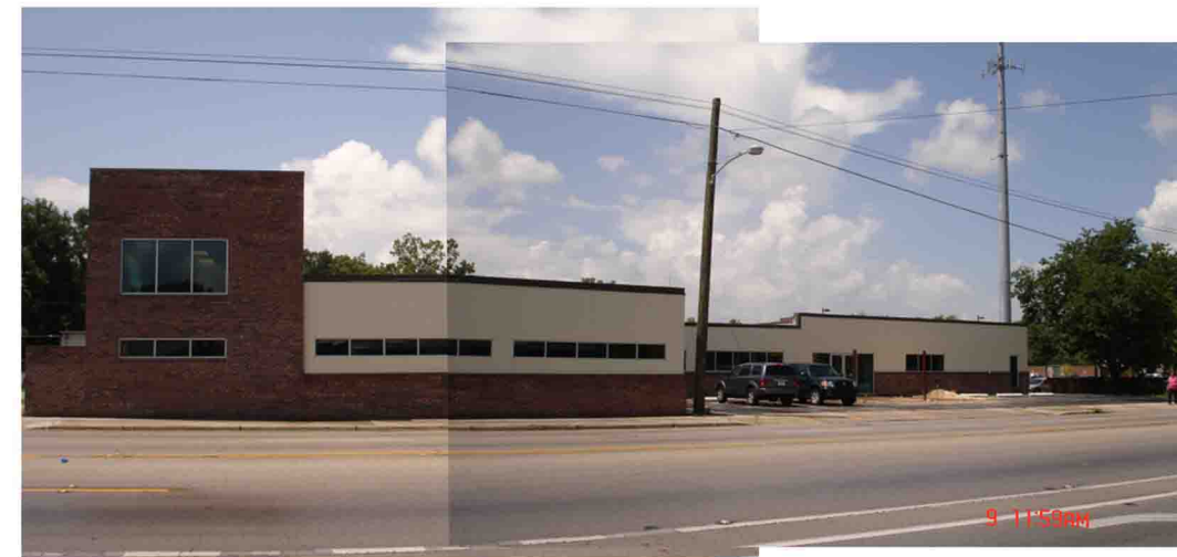
RENOVATED GAINESVILLE PD BUILDING
