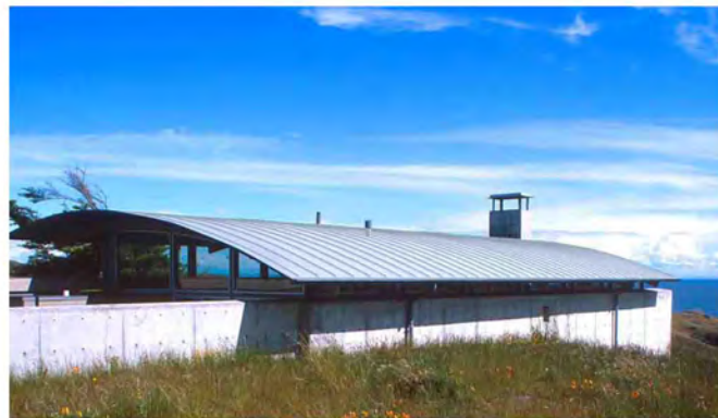
HIGH REFLECTIVITY ROOF SYSTEMS
