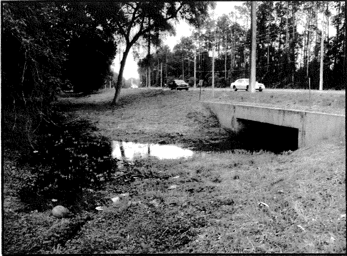
Photo 7. View of the culvert that forms the major hydrologic connection between the project site and areas lying south of NE 39th Avenue.
