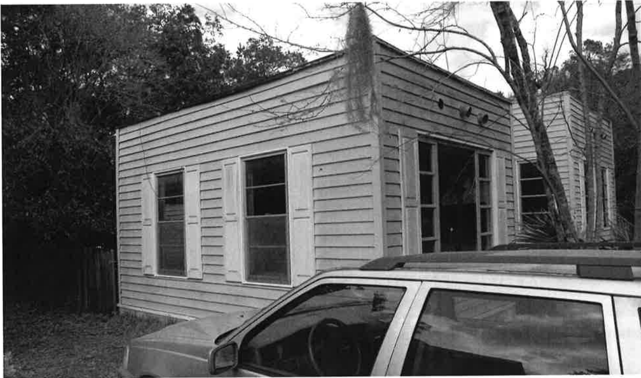
3: South elevation of original carport.
