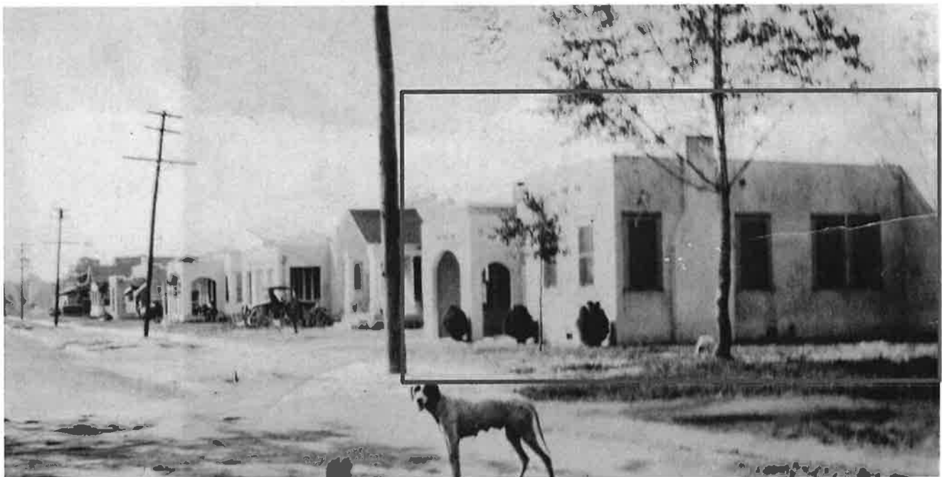
Bottom: Photo c. 1925 showing original house and carport with arched openings. Original windows were wood, with 8/1 sash. Original cladding was stucco.
