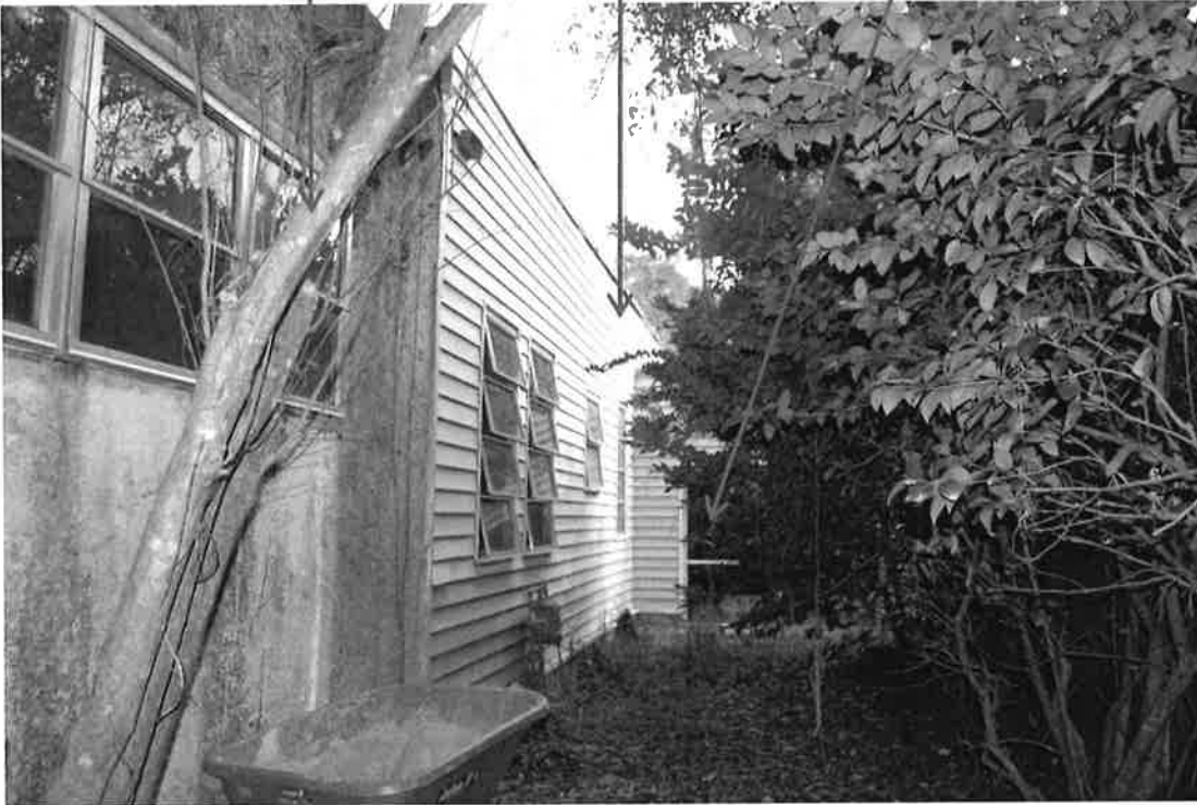
11: Side (south) elevation of master bedroom addition and original house, now clad with siding.
