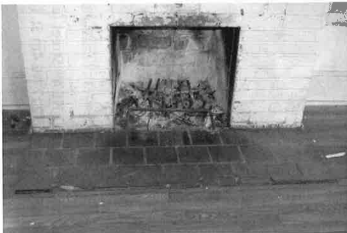
15: Original chimney and fireplace are structurally deteriorated and do not meet code requirements. Chimney is leaning and hearth tile is cracked and sinking.
