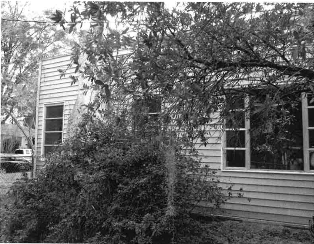
6: North elevation (NE 13 th Avenue) with original chimney and mid-century windows.
