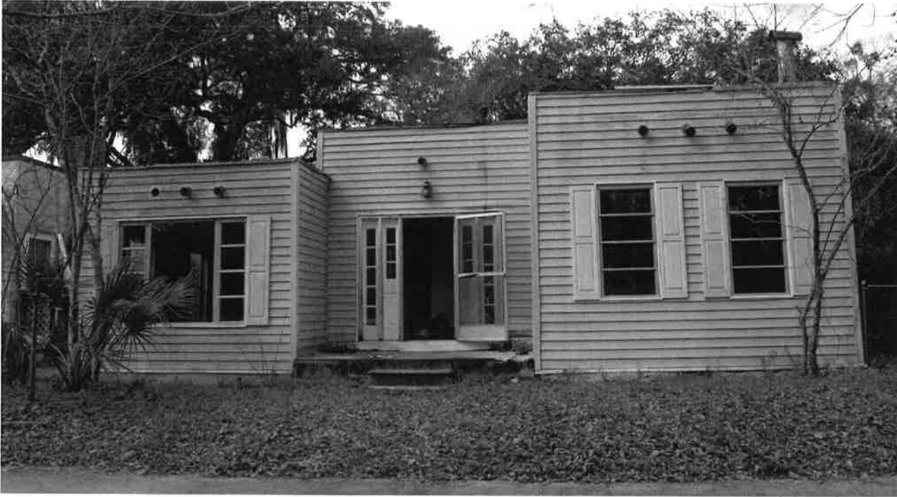
1: Current front façade (NE 4 th Street), showing siding and squared-off modification of front entry opening.
