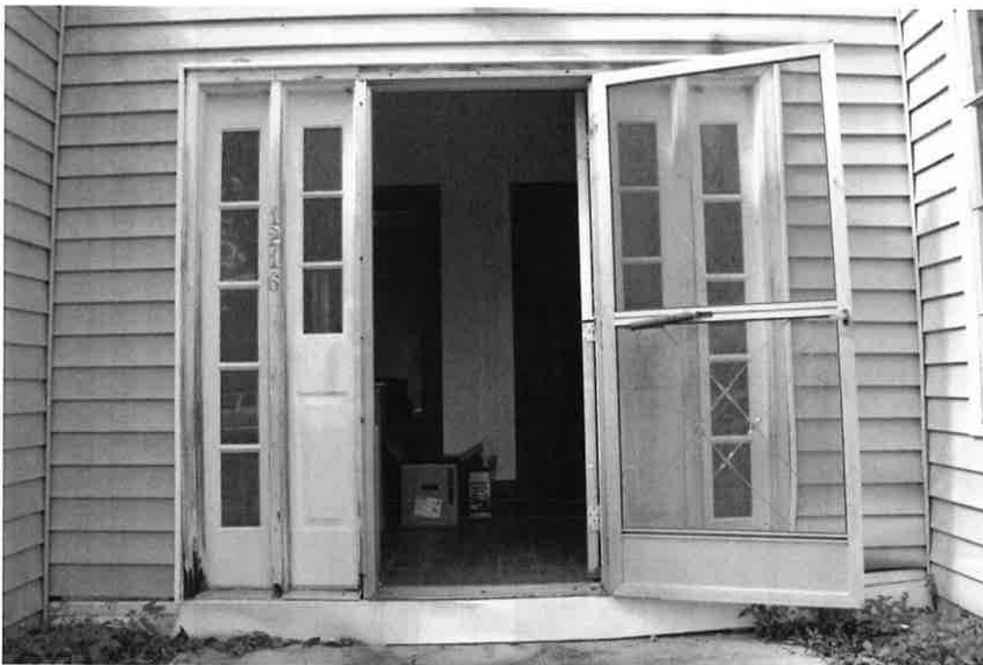
2: The original exterior red porch tile still exists in the current front entryway.
