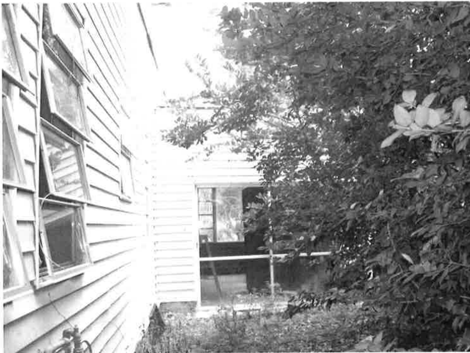
12: Rear (west) elevation of enclosed carport.
