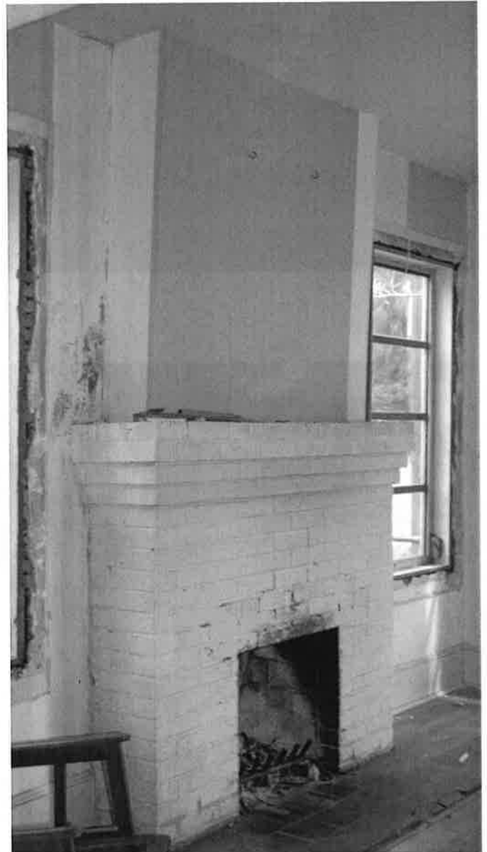
15: Original chimney and fireplace are structurally deteriorated and do not meet code requirements. Chimney is leaning and hearth tile is cracked and sinking.
