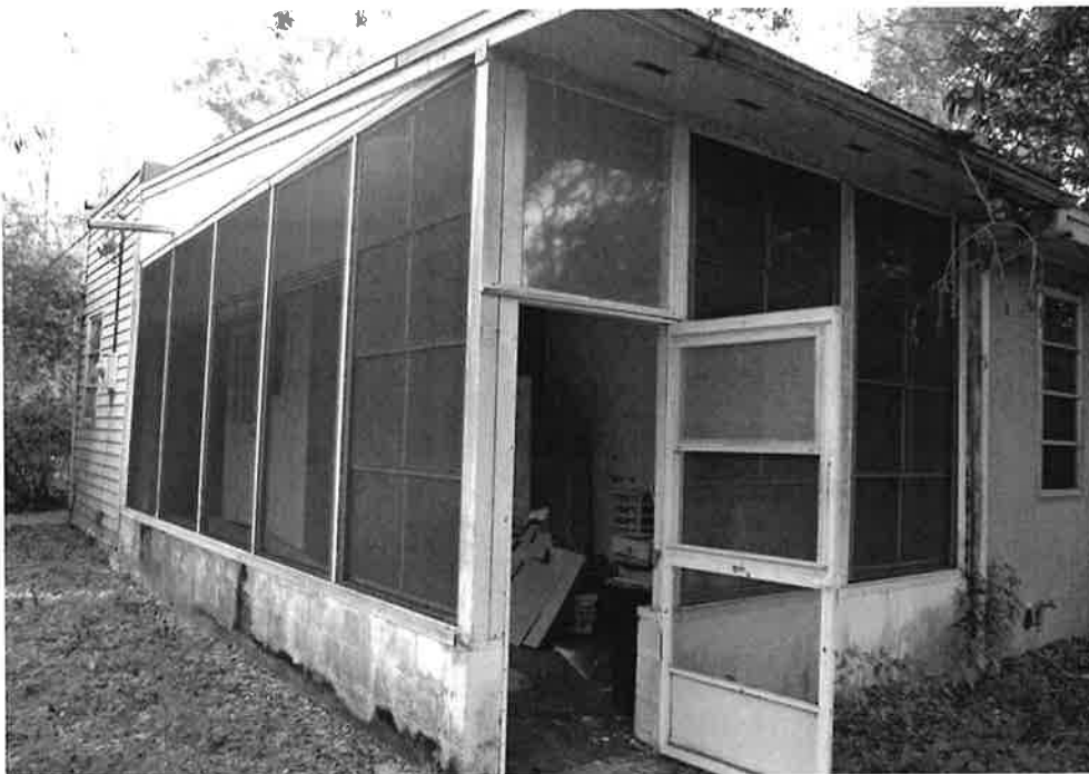
8 (bottom): View of rear porch addition from northwest corner of lot.
