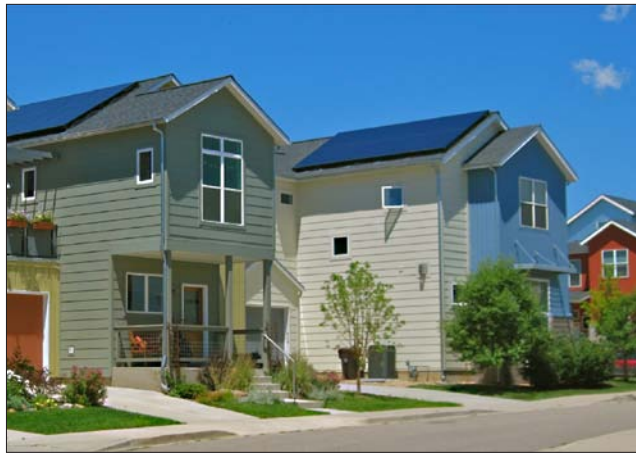
A solar subdivision in Boulder includes IPS solar installations.
