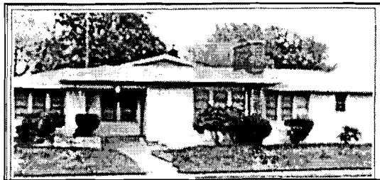
Ranch house (1952) in the Denver Court Historic District, Galveston, Texas. Developed by West Coast architects in the 1930s and promoted by Sunset Magazine in books such as architect Cliff May's Western Ranch Houses (1946), the sprawling Ranch house attained great popularity and appeared nationwide in the 1950s, often on the unbuilt lots of early subdivisions. (Photo by Lesley Sommer, courtesy Texas Historical Commission)
