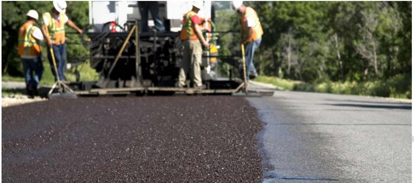
Figure 4. Crew Applying a Microsurfacing Treatment to Crack Sealed Asphalt Pavement
