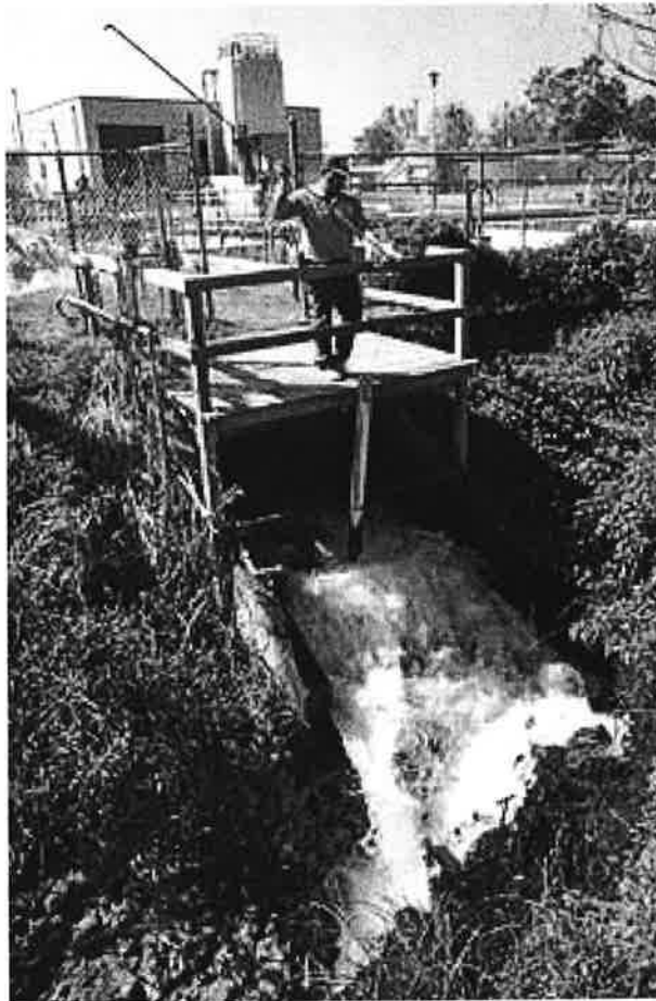
The Gainesville Regional Utilities Main Street Wastewater Treatment Plant daily discharges about 6 million gallons of treated effluent into Sweetwater Branch, which flows onto Paynes Prairie and into Alachua Sink. JOHN MORAN/The Gainesville Sun
