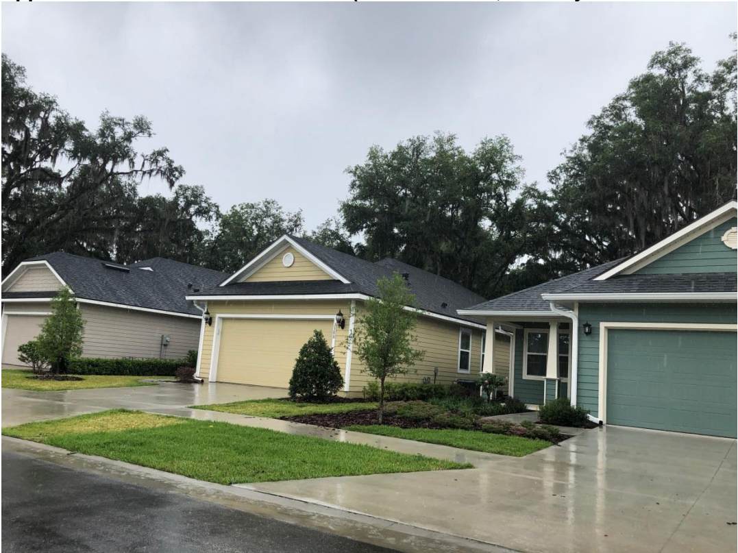
Appendix C.4 Walnut Creek Phase II (Southern Area; No alley or service easement)
