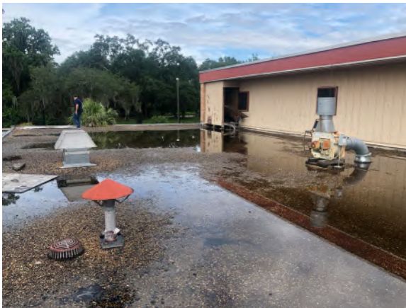
Figures: Built-up-roof (BUR) and standing water. Despite the drain located in the lower left corner of the left photo, there is insufficient slope for draining excess water.
