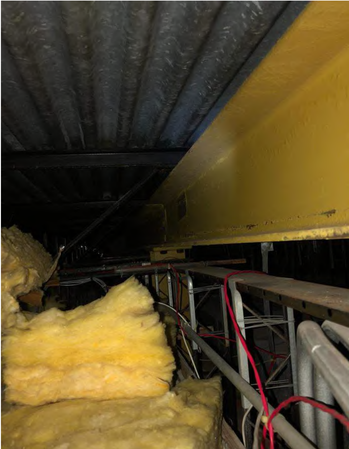
IMAGE 7: ROOF STEEL BEAM OVER STEEL COLUMN
