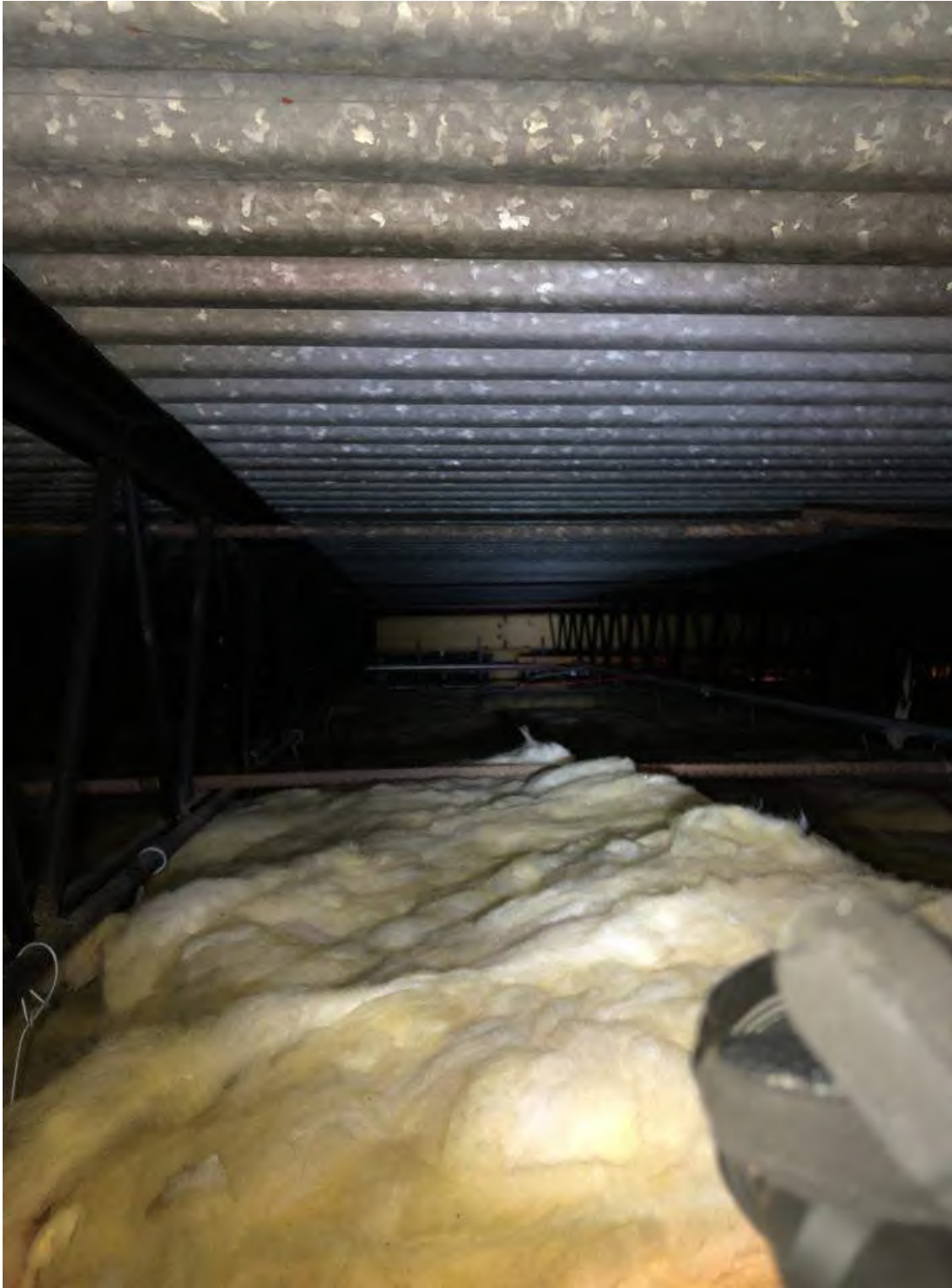
IMAGE 6: ROOF AND JOISTS OVER APPARTUS BAY
