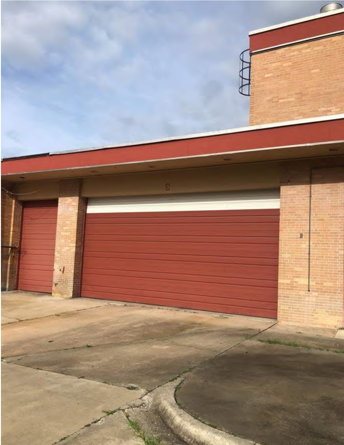
IMAGE 11: EAST EXTERIOR FACE OF BUILDING
