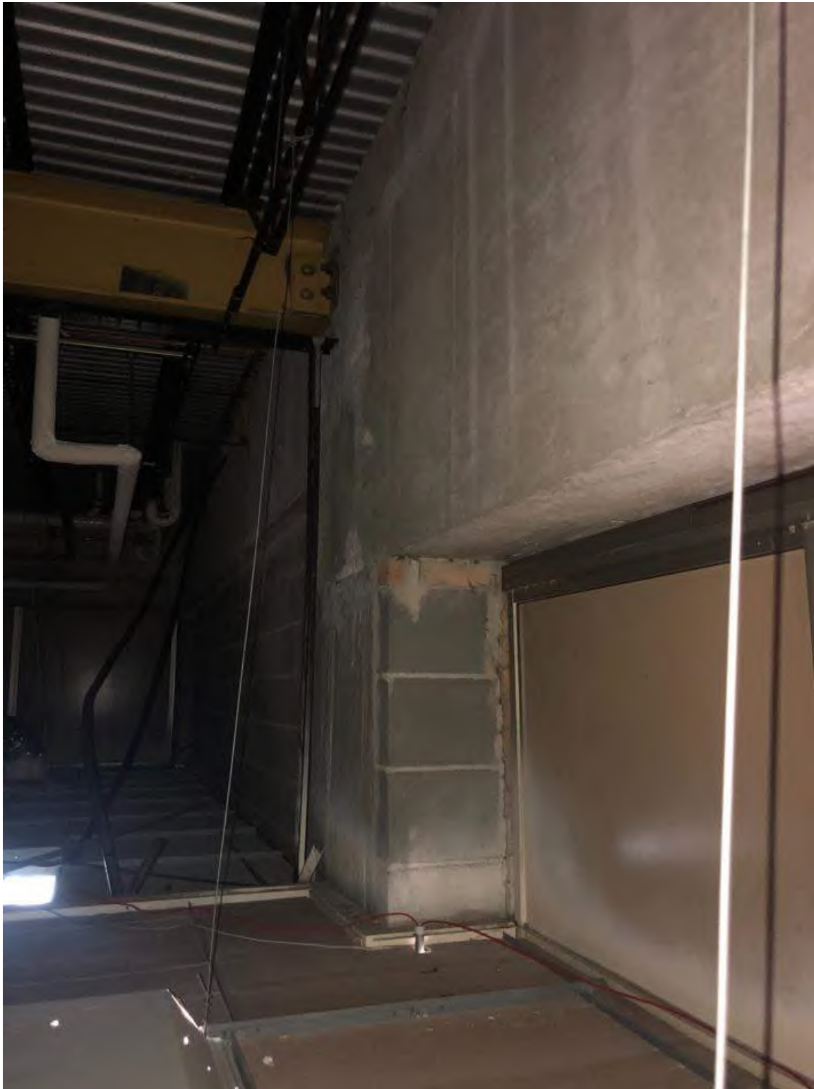
IMAGE 3: CMU WALL WITH PERIMETER CONC BEAM
