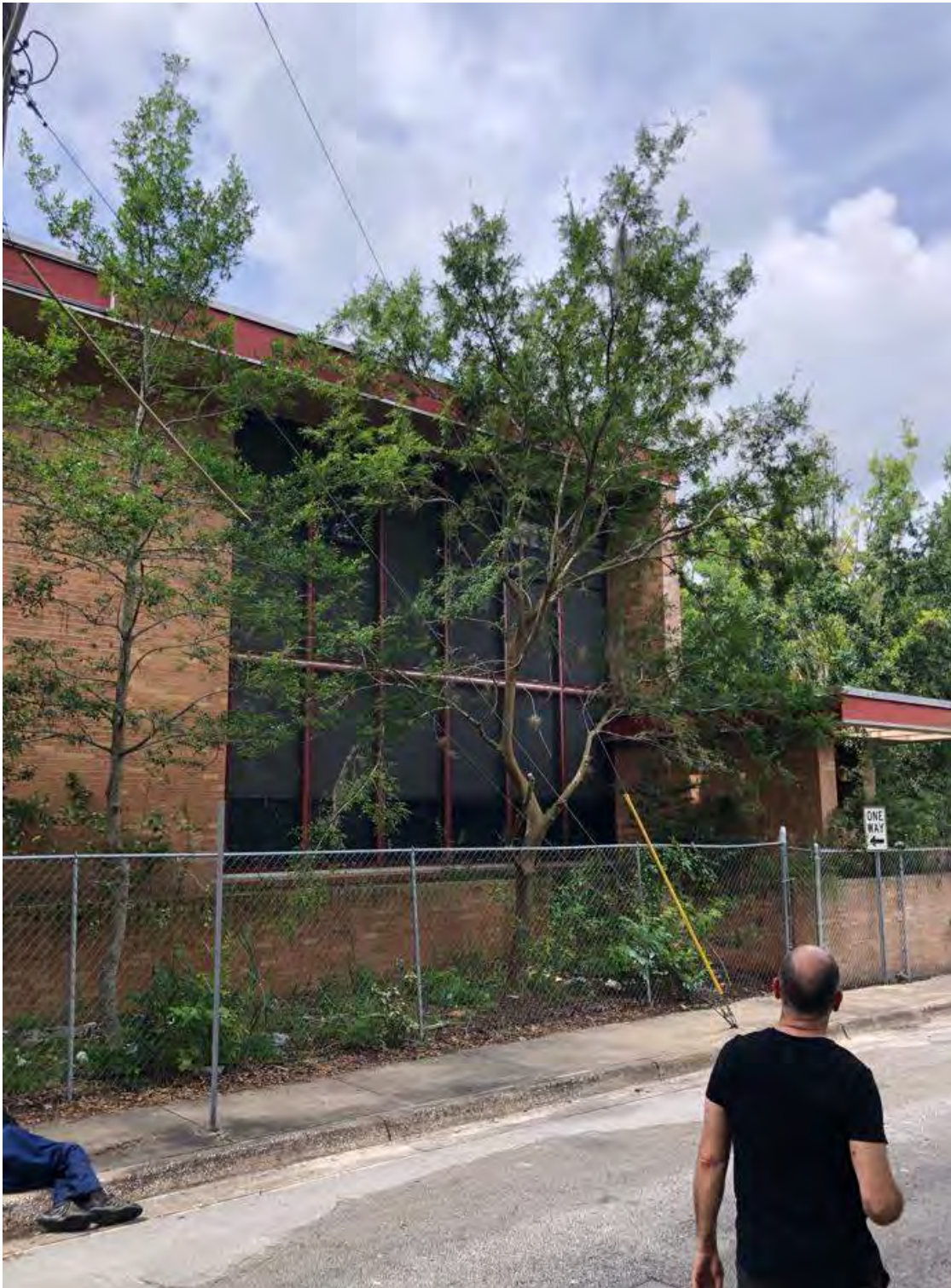
IMAGE 13: NORTH EXTERIOR FACE OF BUILDING
