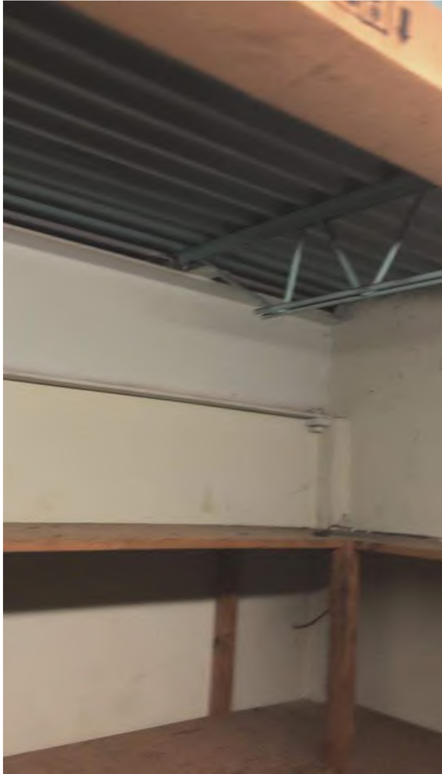
IMAGE 10: STEEL JOIST ON STEEL GIRDER BETWEEN APPARATUS BAY AND STORAGE ROOM
