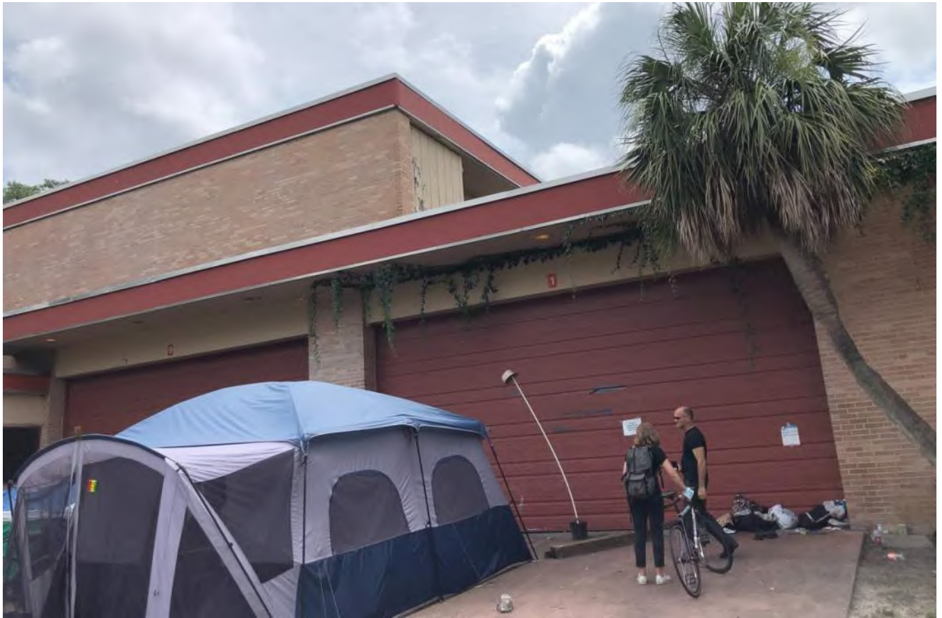
IMAGE 12: WEST EXTERIOR FACE OF BUILDING
