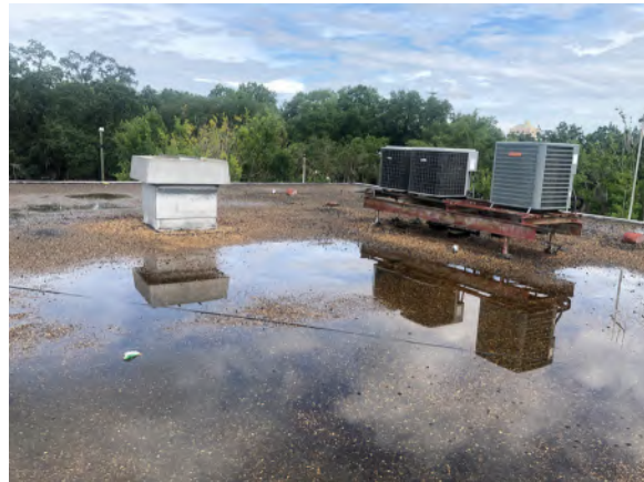
Figures: Built-up-roof (BUR) and standing water. Despite the drain located in the lower left corner of the left photo, there is insufficient slope for draining excess water.
