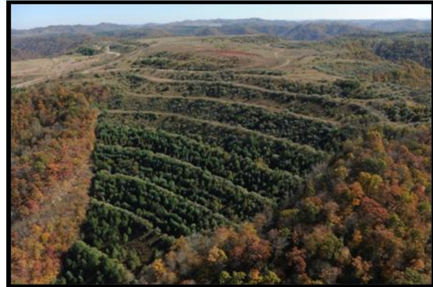
Valley fill located off of the Twisted Gun Golf Course located in Mingo County, West Virginia
