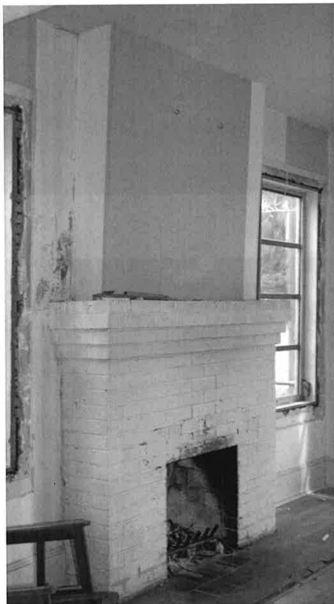
15: Original chimney and fireplace are structurally deteriorated and do not meet code requirements. Chimney is leaning and hearth tile is cracked and sinking.
