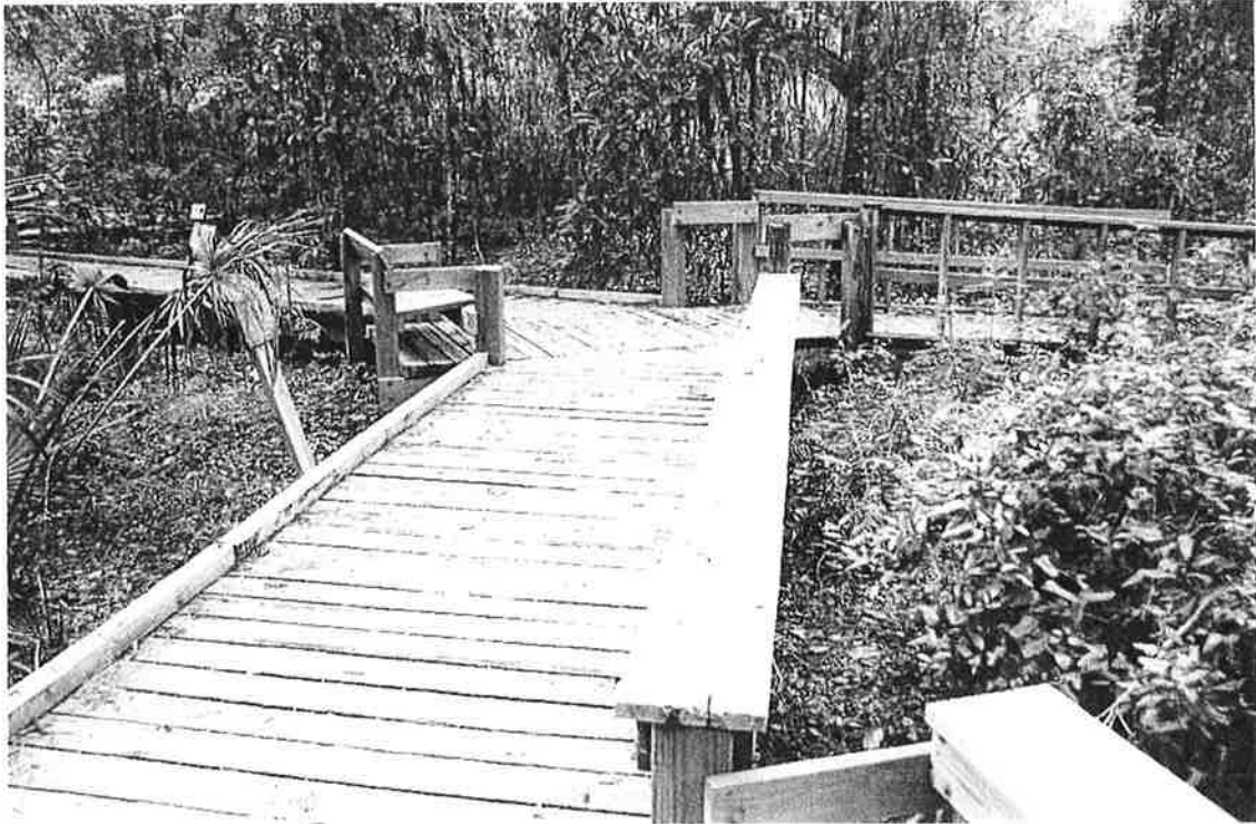
TYPICAL VIEW OF BOARDWALK
