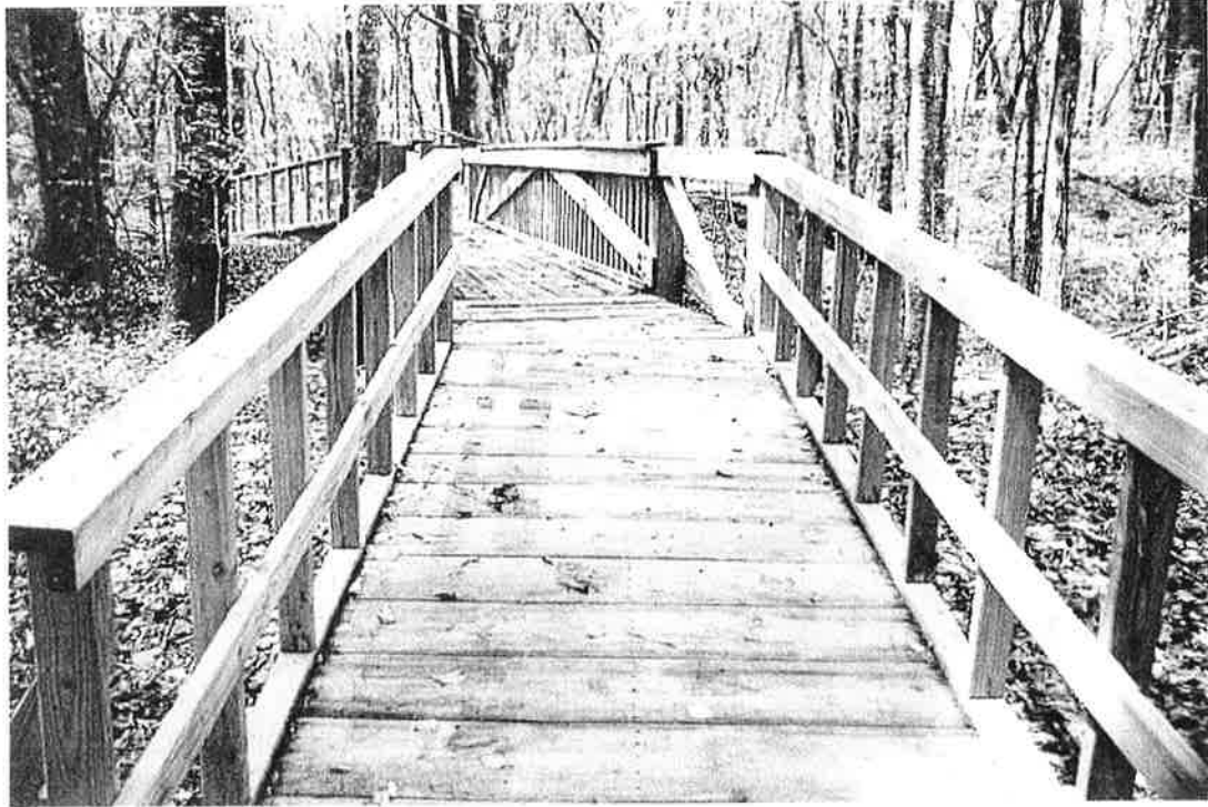
RECENTLY REPAIRED BOARDWALK
