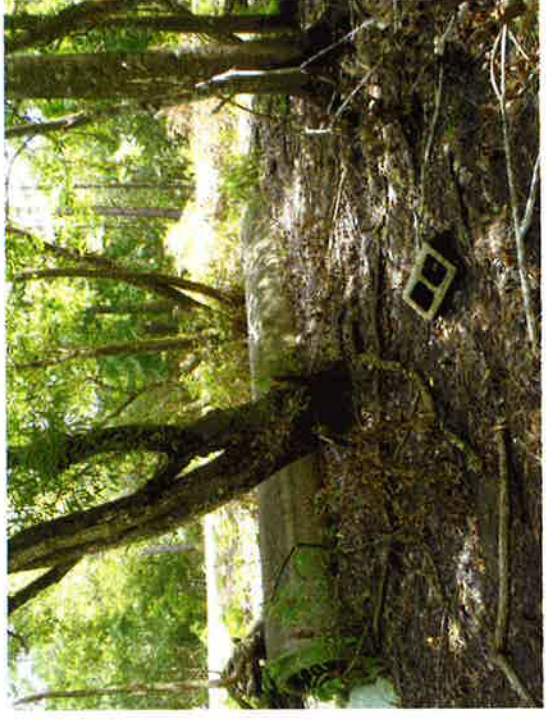
(d) Effluent culvert located on downstream side of structure
