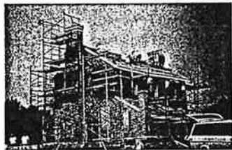
Matthew Jones House restoration
