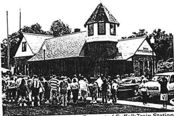
Opening Day at the Renovated Suffolk Train Station, Suffolk, Virginia
