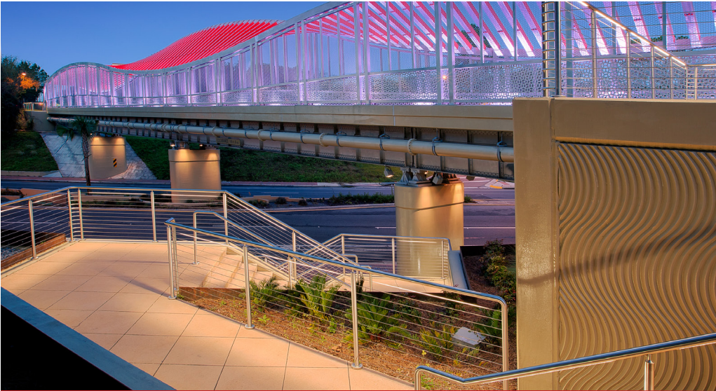
At SW 13th Street, we implemented measures that involved recycling materials such as concrete and choosing sustainable products and systems.
