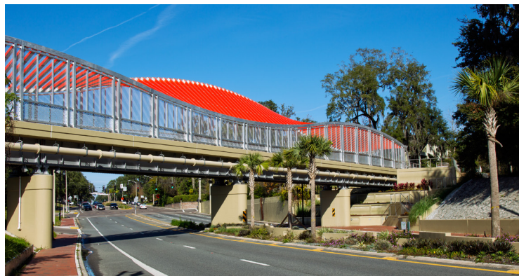
2014 APWA National and State Project of the Year for Structures under $5 Million
