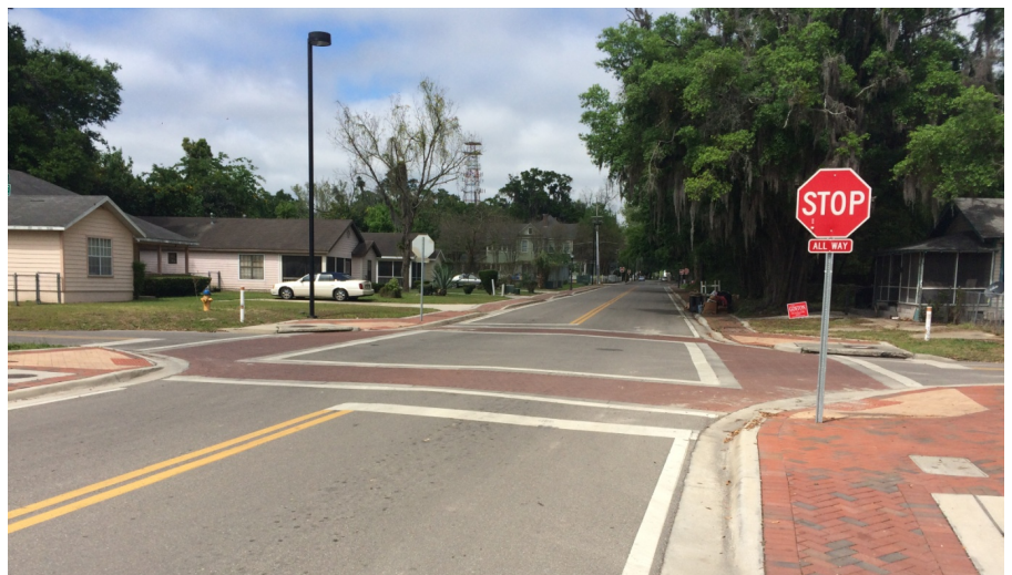
For the CRA's SW 3rd Avenue streetscape, project manager Derek Dykes scheduled lane closings during low traffic times to lessen the impact on the surrounding community while milling and refinishing the roadway.
