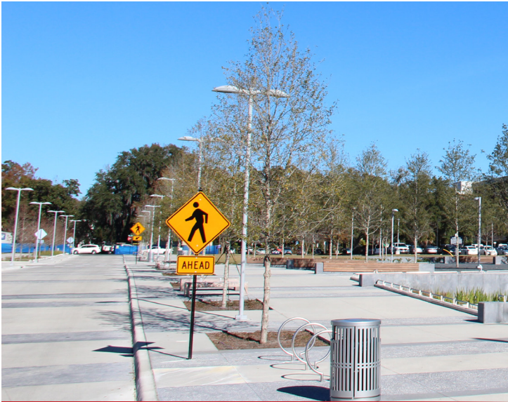
SW 9th Street features accommodations for pedestrians, cyclists, and motorists, with a focus on safety for everyone.
