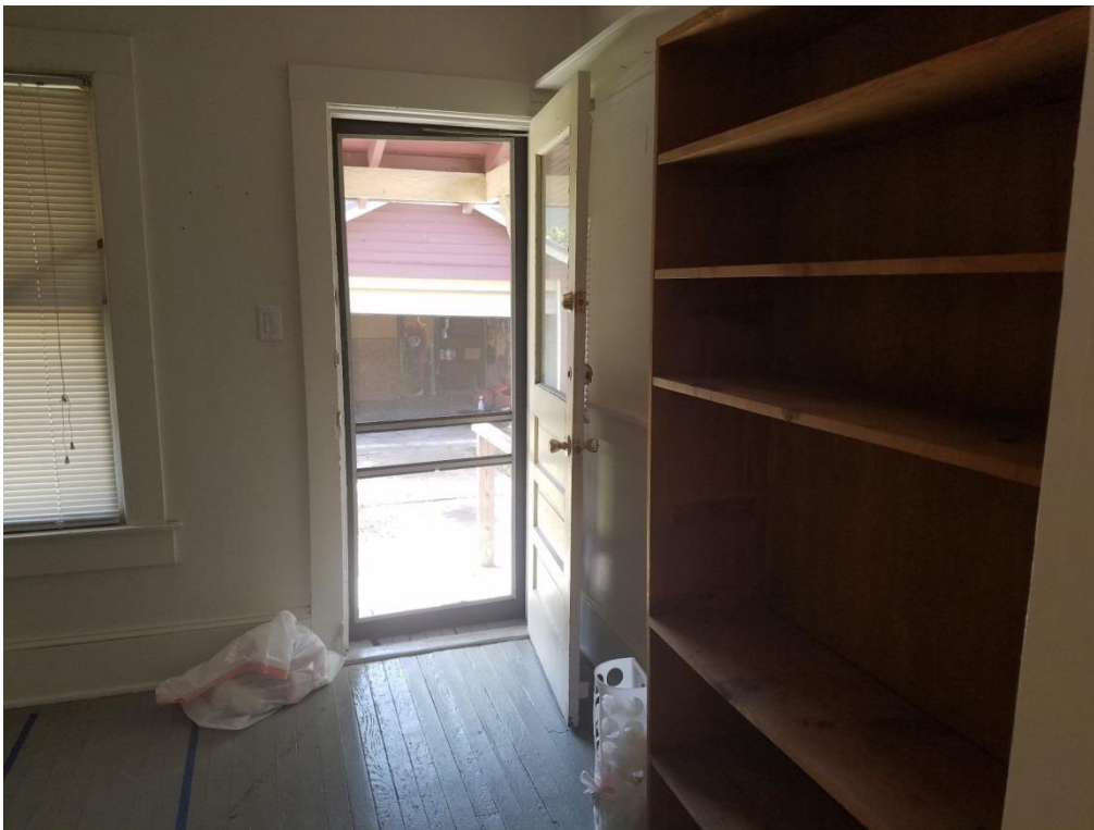
Kitchen: view of north wall with windows (top)
