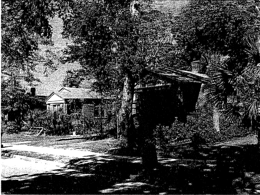
Existing 1928 Bungalows, looking NE
