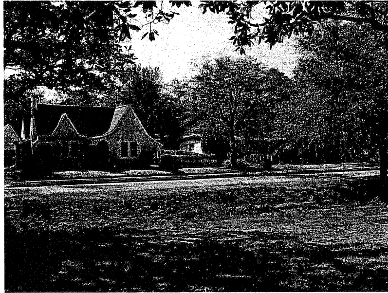
Looking SW from the project site.
