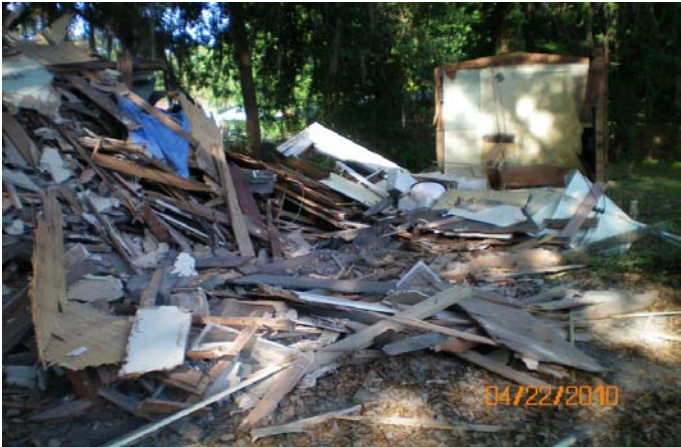
House Reconstruction- During (Demolished)
