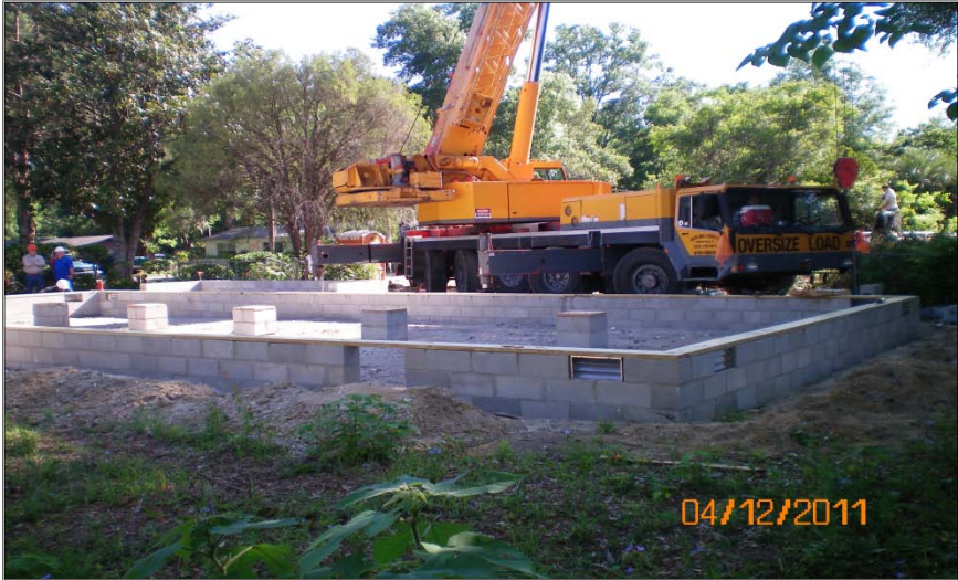
New Construction-Infill Housing (The Foundation)
