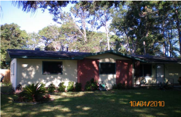
Roof Program- Roof Replacement (Before)
