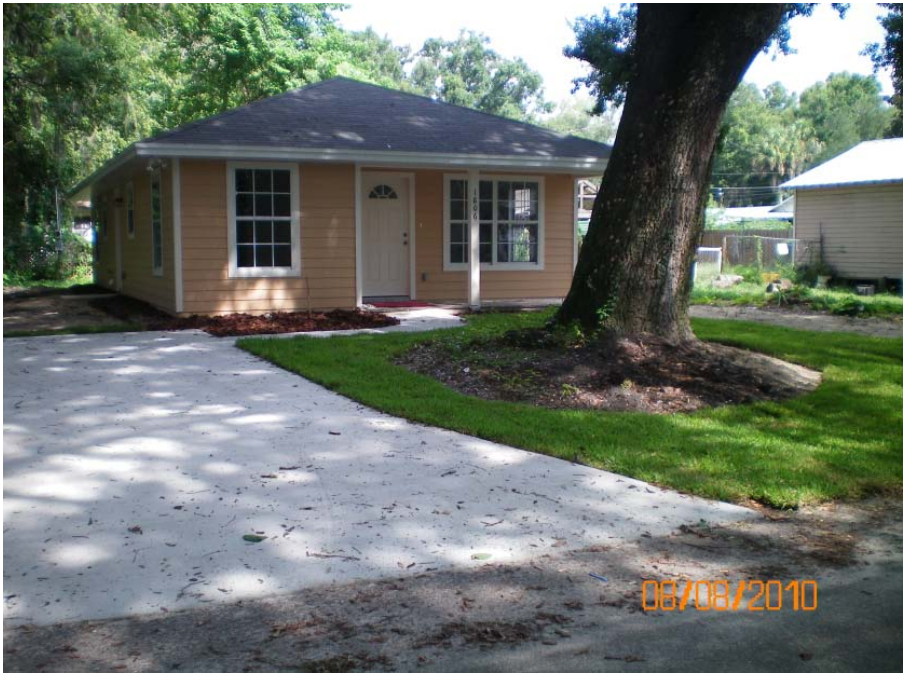
House Reconstruction Program – After
