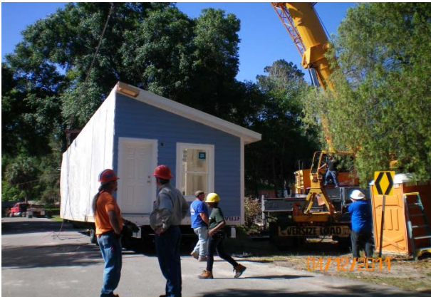
New Construction-Infill Housing (Side Two Lifted)
