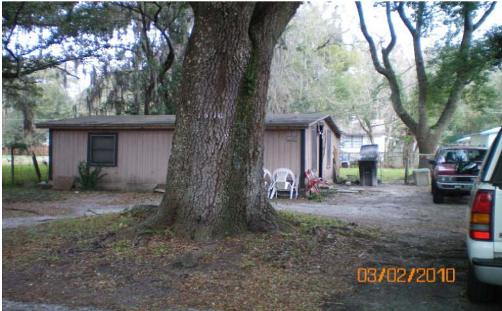
House Reconstruction- Before
