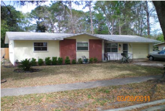
Roof Program- Roof Replacement (After)
