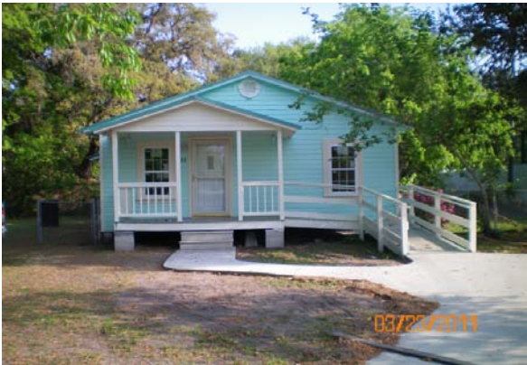
Housing Rehabilitation- After
