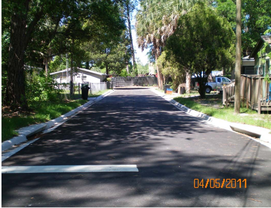
Public Infrastructure- Duval Area Neighborhood
