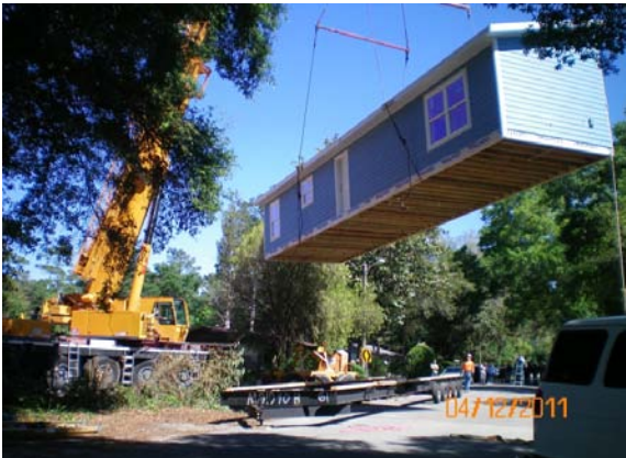
New Construction-Infill Housing (Side One Lifted)
