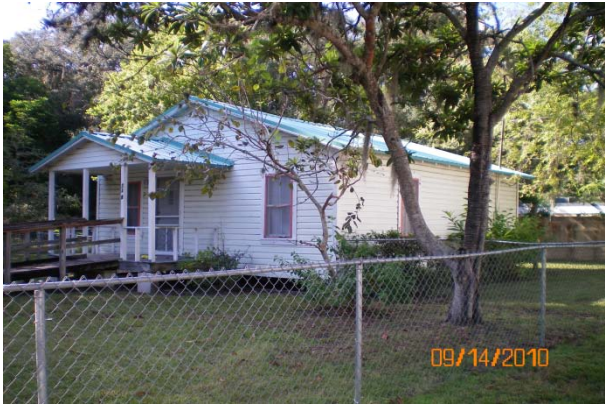
Housing Rehabilitation- Before
