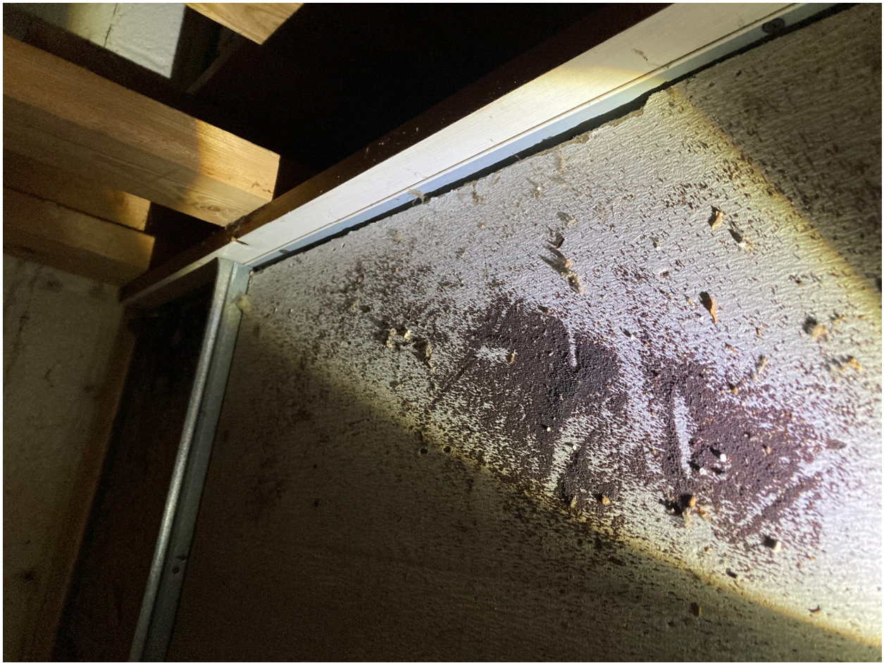
Figure 9. Example of black pellets from suspected termites on suspended ceiling added during 1990's renovation.
