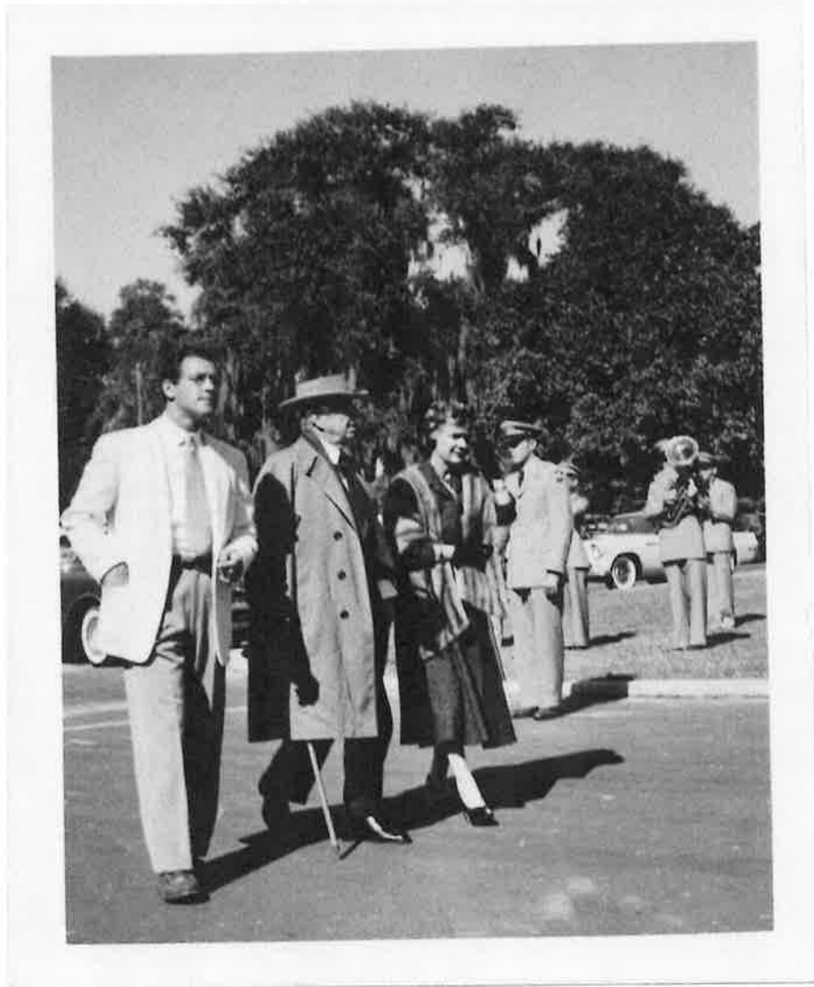
Inspection of Polk County Science Building, November 4, 1955, Lakeland, Florida.
