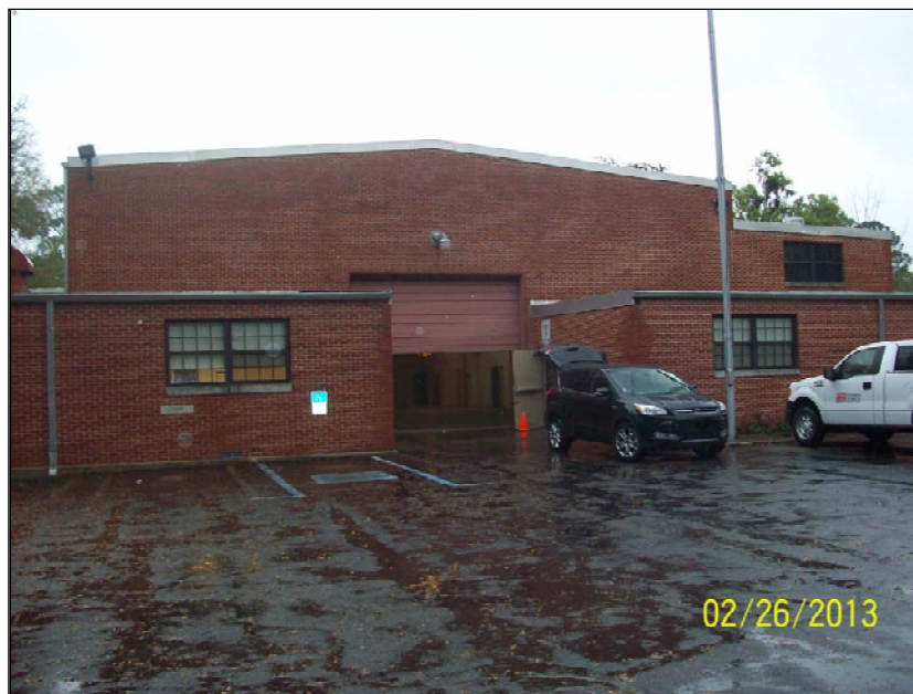
Photo 1: Front of USARC Building. Confirmed ACM: roof flashing material
