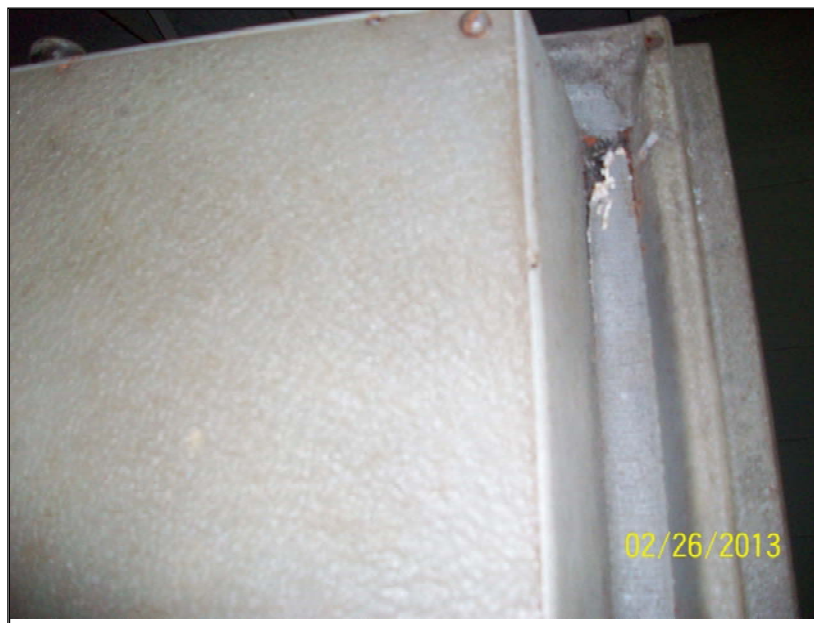
Photo 8: Confirmed ACM: woven gasket adhered to the seal of the arms vault door
