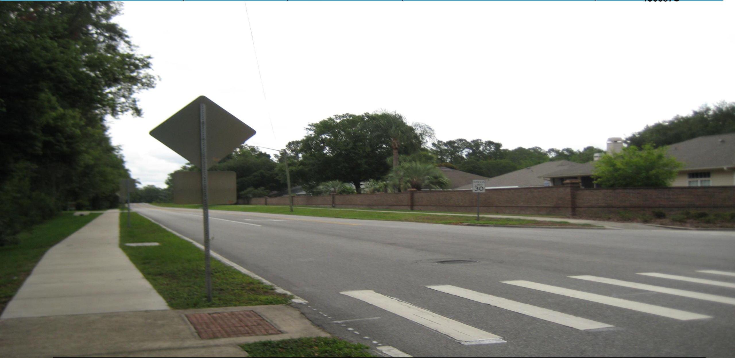
View of Sterling Place on NW 73 rd Avenue Looking East
