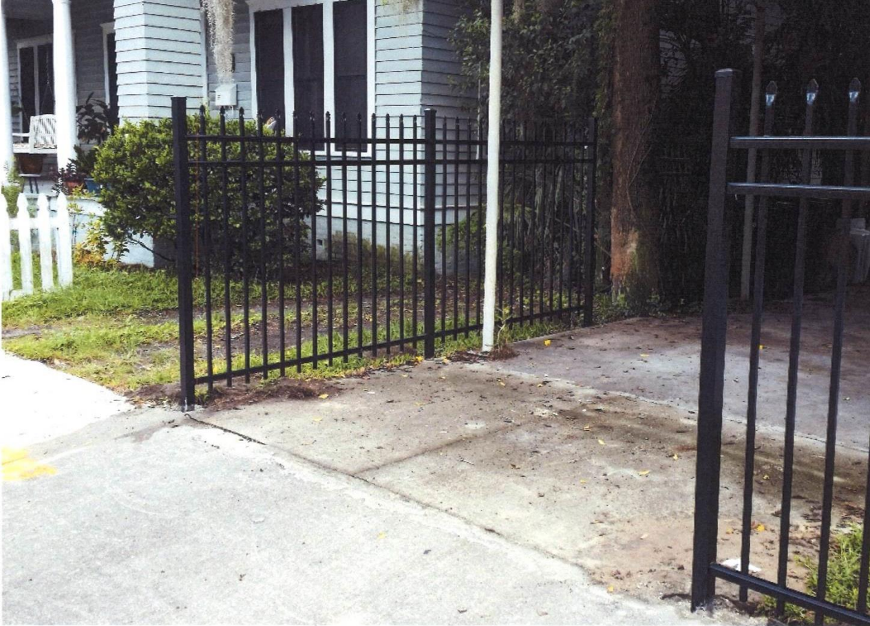
Fencing adjacent to existing driveway, no gate.
