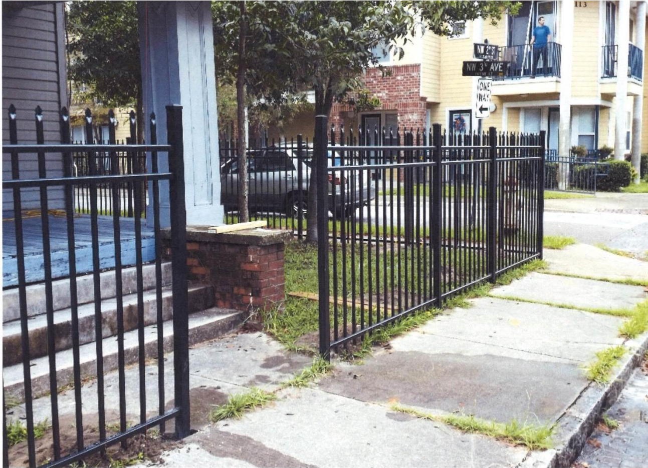
Fencing at front walkway, no gate.
