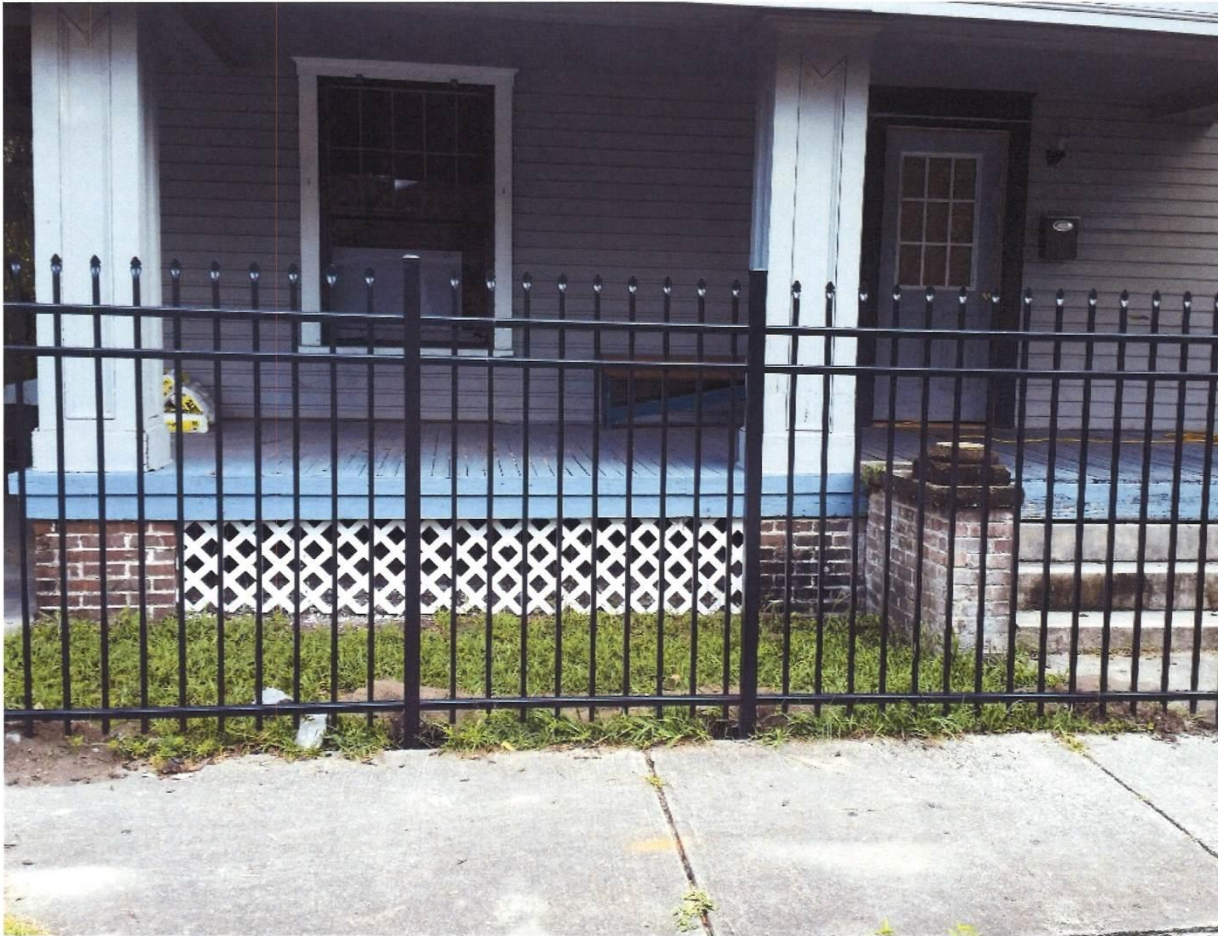
Details of the installed fence.
