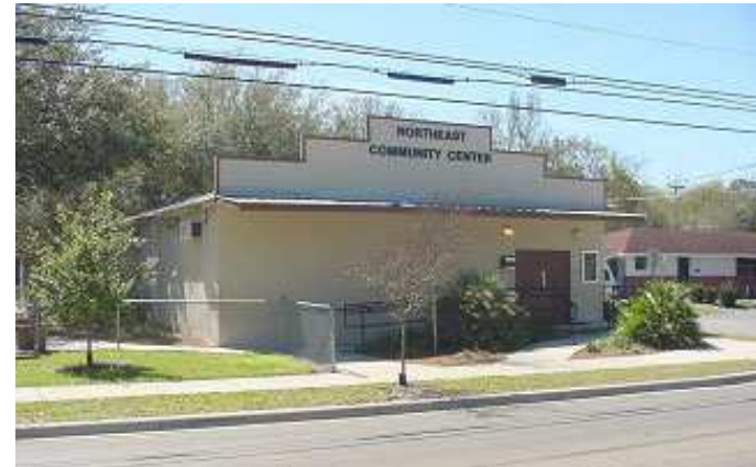
Northeast Community Center
