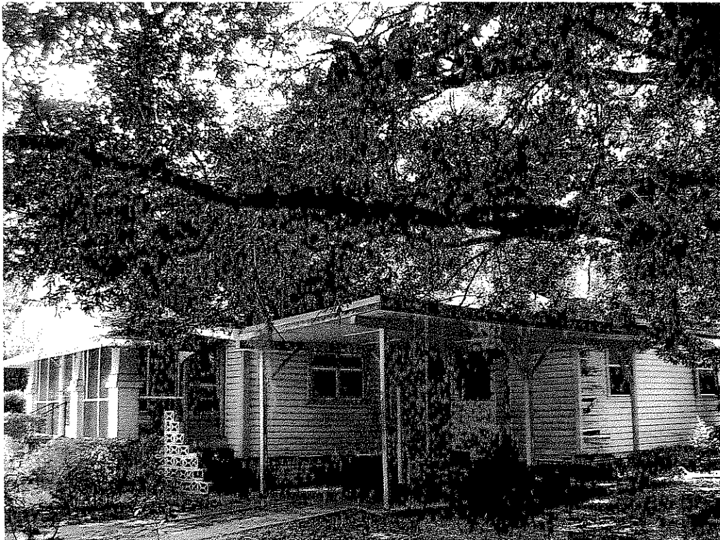
Photograph 6: West façade, showing carport, facing southeast.
