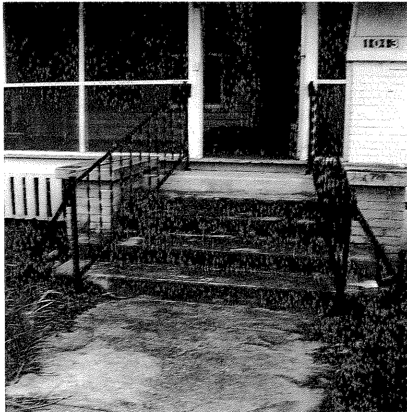
Photograph 8: Front steps, facing south.
