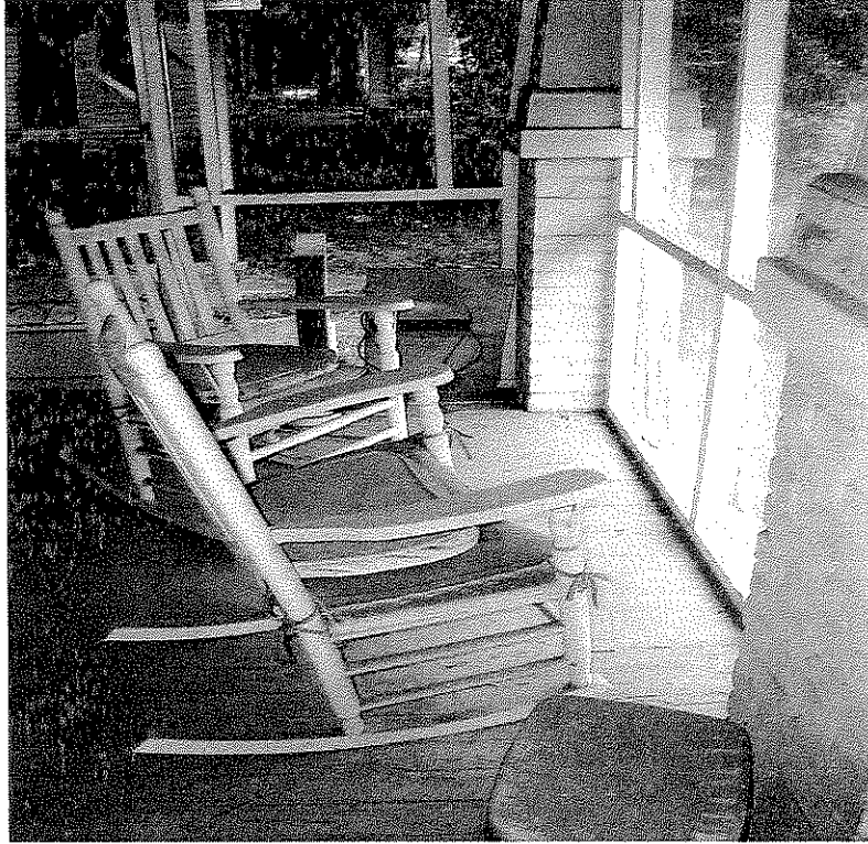
Photograph 7: Front porch, facing west.
