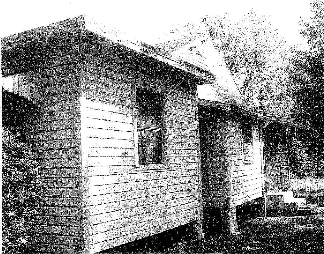
Photograph 5: South, rear façade, facing northeast
