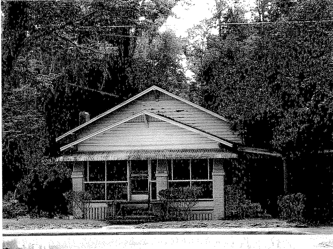
Photograph 1: Front façade, facing north: SOUTH
