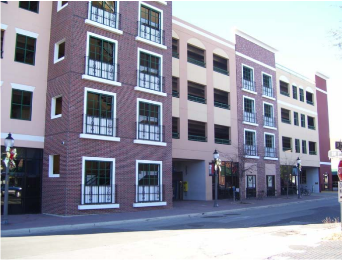
City Parking Garage
