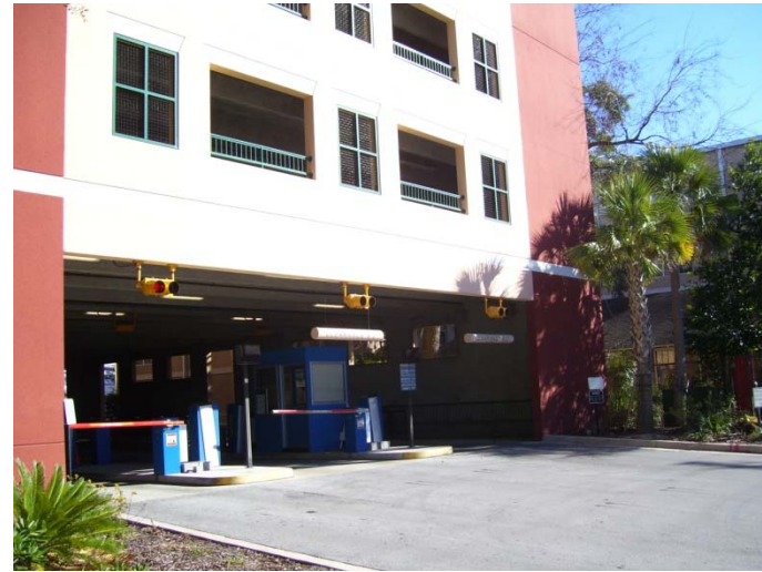
City Parking Garage
