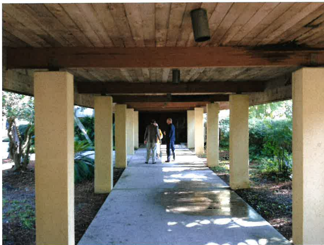
View under breezeway (Photo: Mikesch Muecke)
