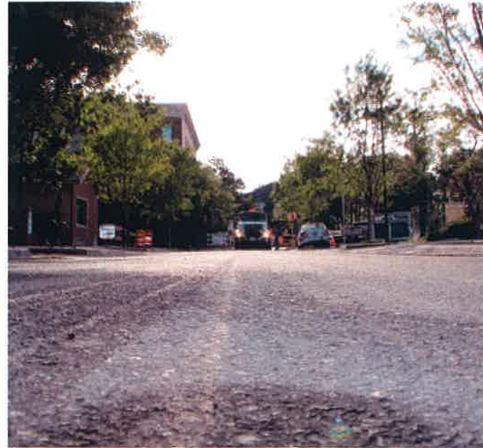
An asphalt truck mobilizes in preparation for the final layer.
