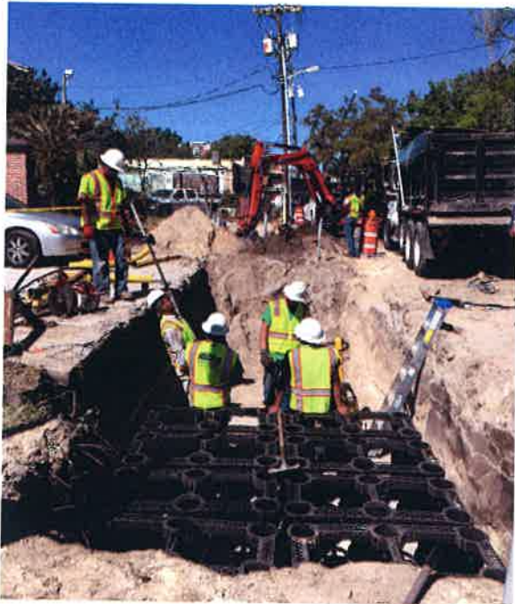
Silva Cell installation.
