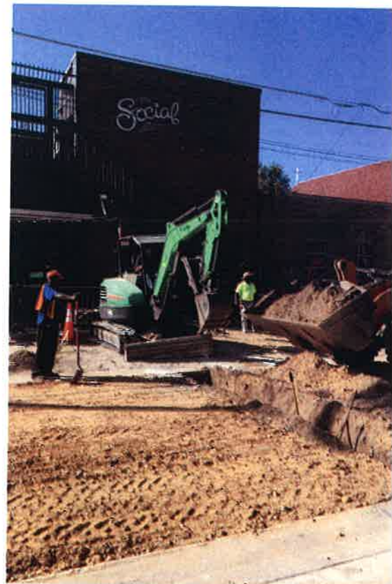
Preparations for street paving.
