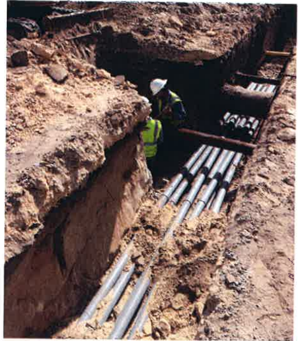
Joint utility trench installation.
