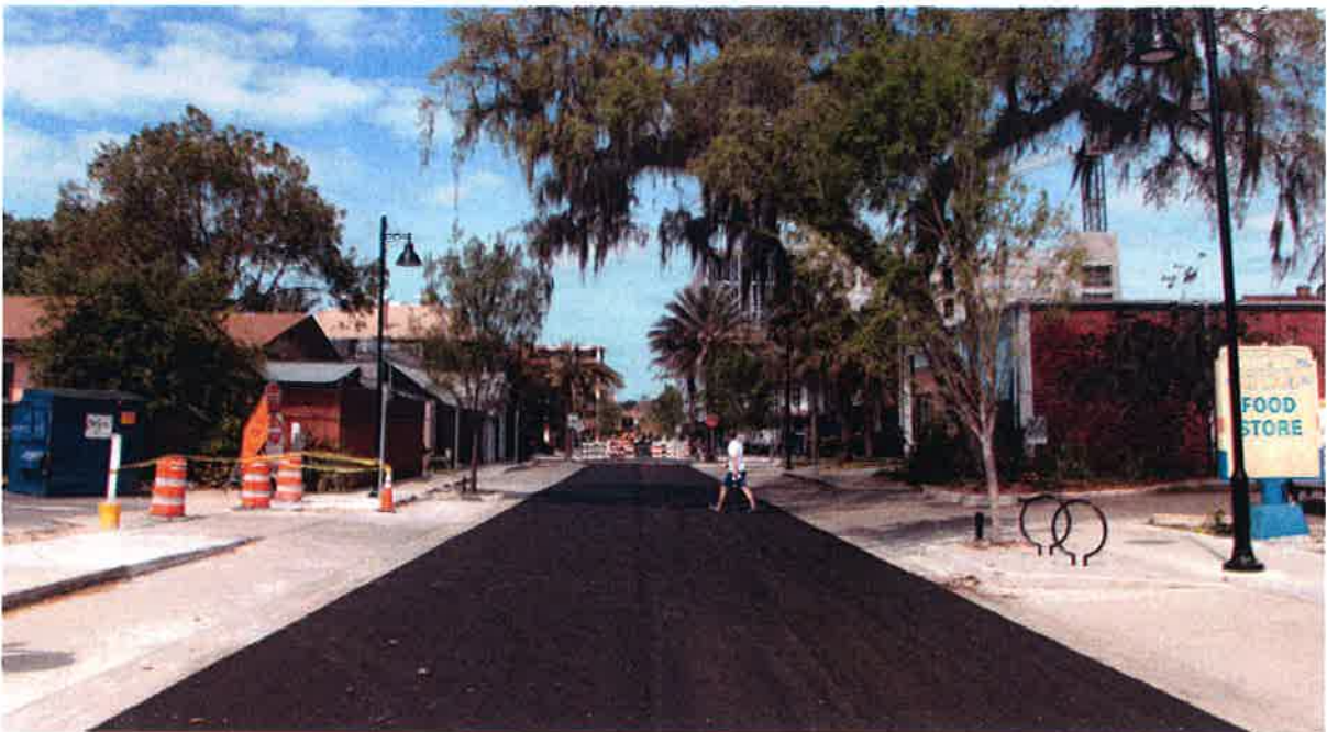
The final layer of asphalt.
