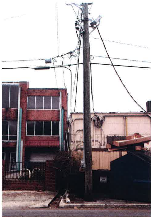
Utility poles and overhead wires interrupted the sight line.
