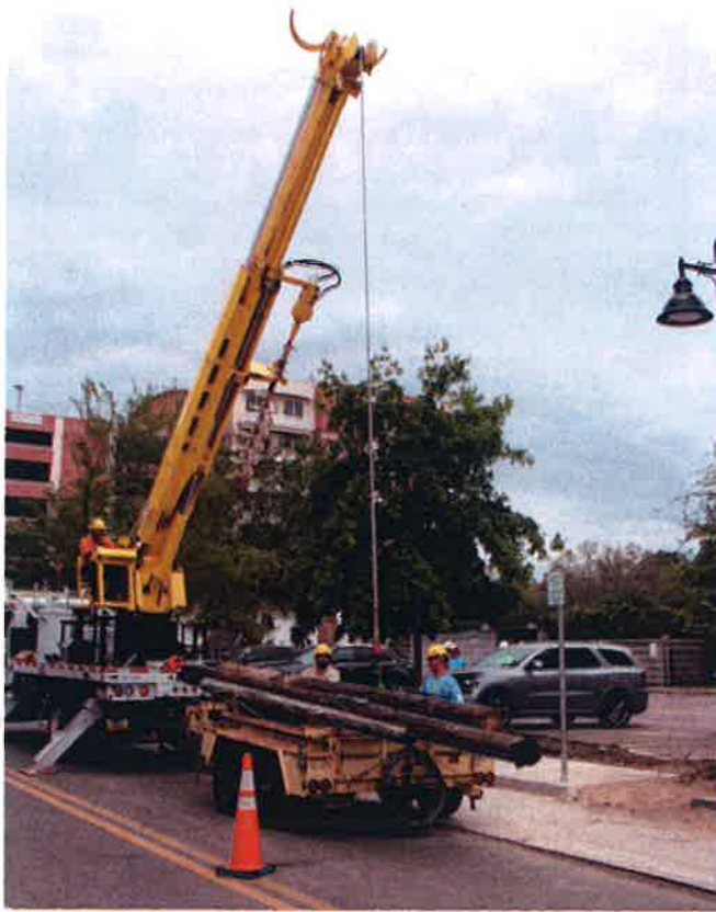
Crews removing the final utility pole.
