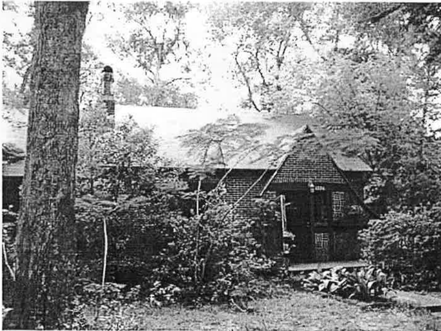
1226 NW 4 th Avenue North University District
