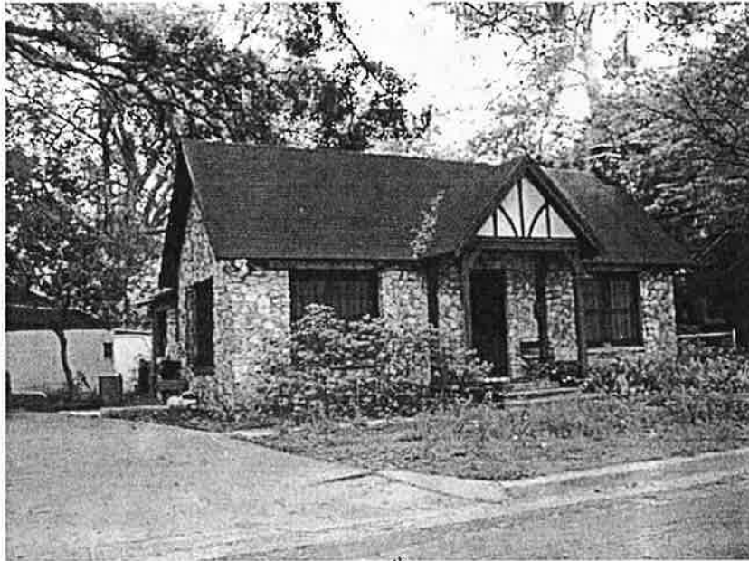
1215 NW 4 th Avenue North University District
