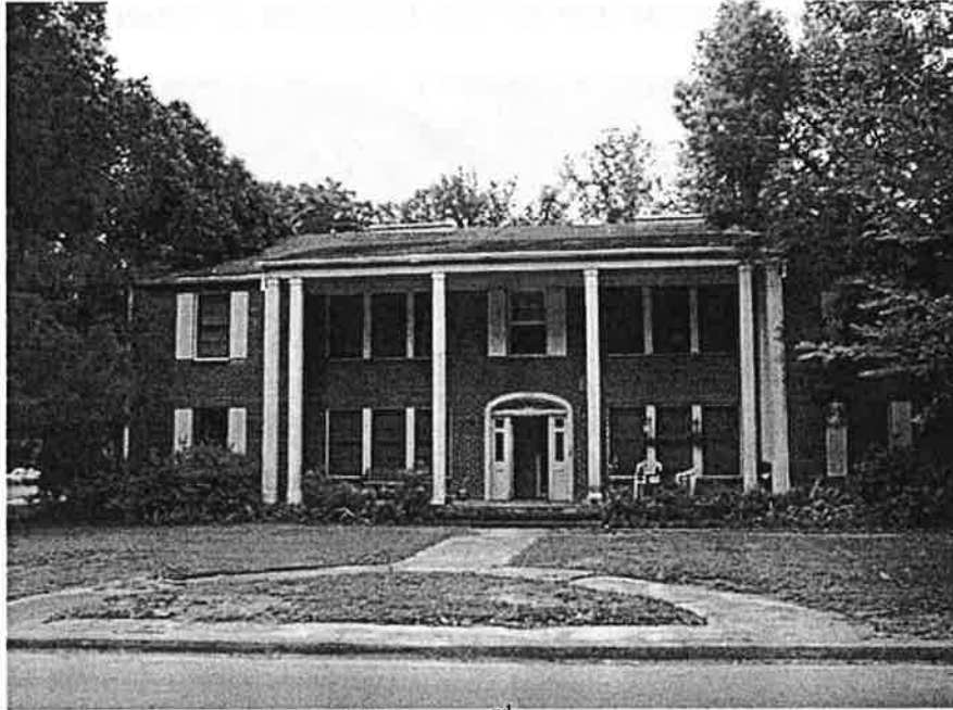
1105 SW 3 rd Avenue South University Avenue
