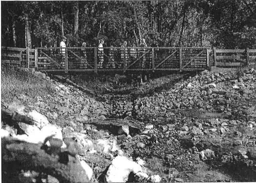
Judy Broward leads a tour group across a newly built bridge spanning Beville Creek during the Cofrin Nature Park Celebration on Tuesday. PHOTOS BY ROB C. WITZEL/STAFF PHOTOGRAPHER
