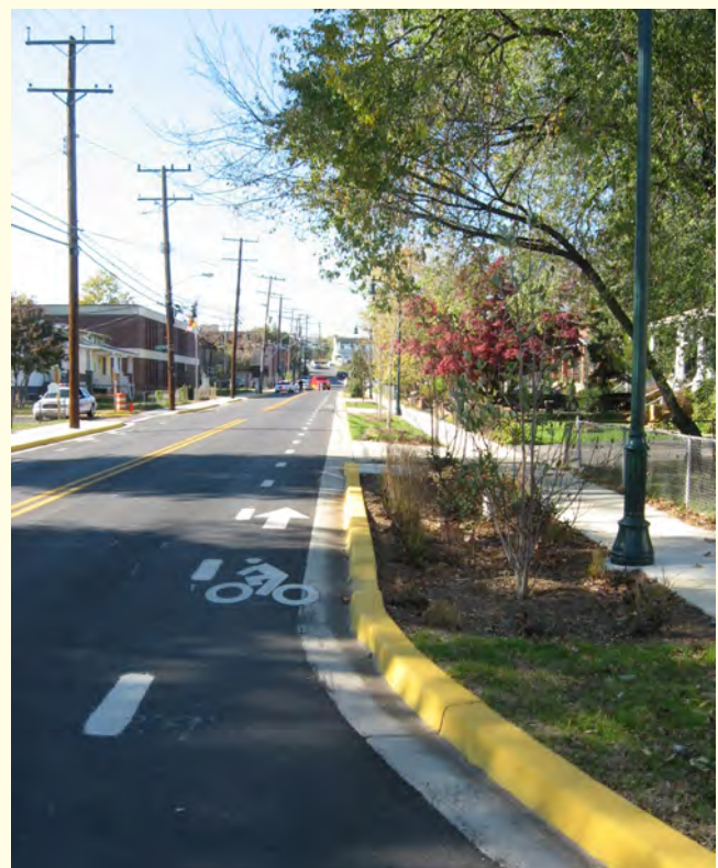
Decatur Street's bike lanes are constructed with permeable materials that allow water to filter through instead of collecting on top. Photo courtesy of Faith Cole.
