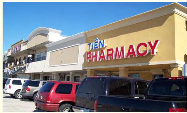
The Mary Queen of Vietnam Community Development Corporation's Façade Improvement Program supported the construction of business plazas and new façades for local establishments. Photo courtesy of Mary Queen of Vietnam Community Development Corporation.
