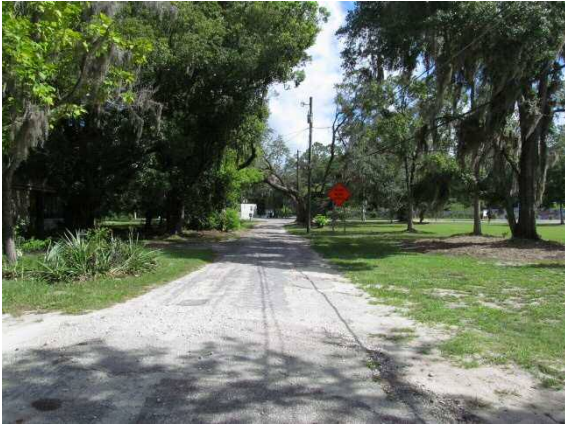
SE 21 st street facing north
