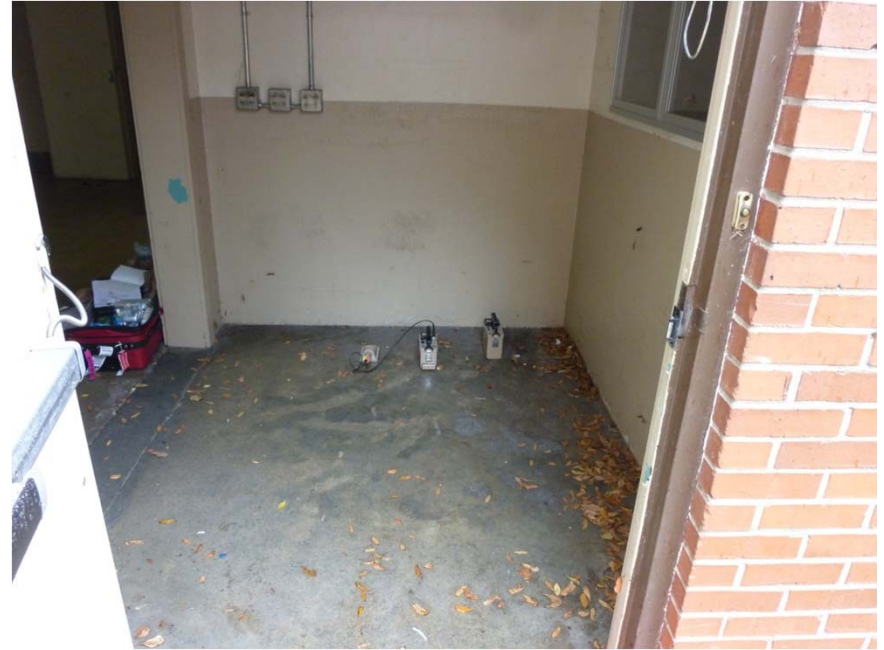
Layton USARC_Background entryway near rollup door
