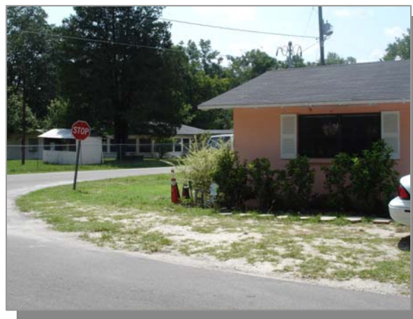
Figure 3.17: Sample of Code Violation: cited as a dangerous building.
