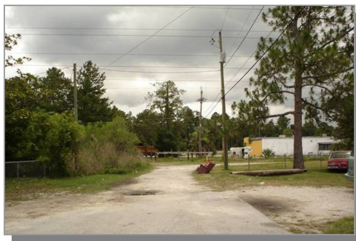
Figure 3.3: Example of a partially unpaved roadway that lacks adequate drainage and pedestrian facilities.
