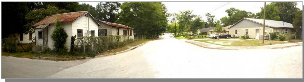
Figure 3.13: New construction adjacent to deteriorated housing.
