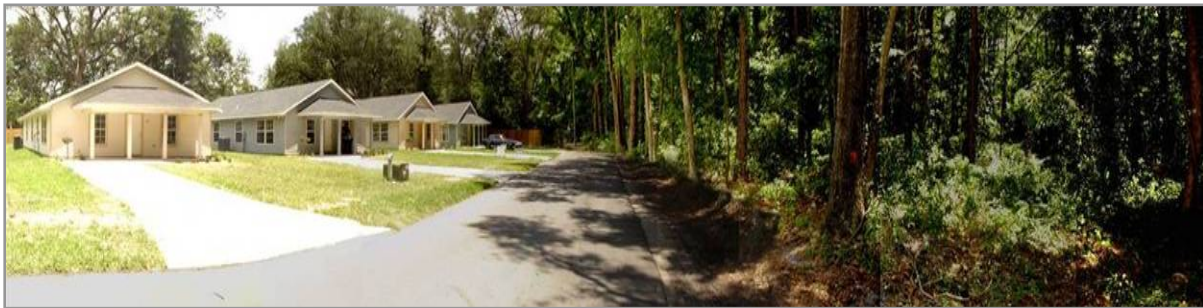
Figure 3.9: New Construction Adjacent to Undeveloped Land
