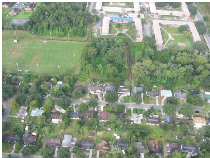
Figure 3.14: Aerial of Kennedy Homes property
