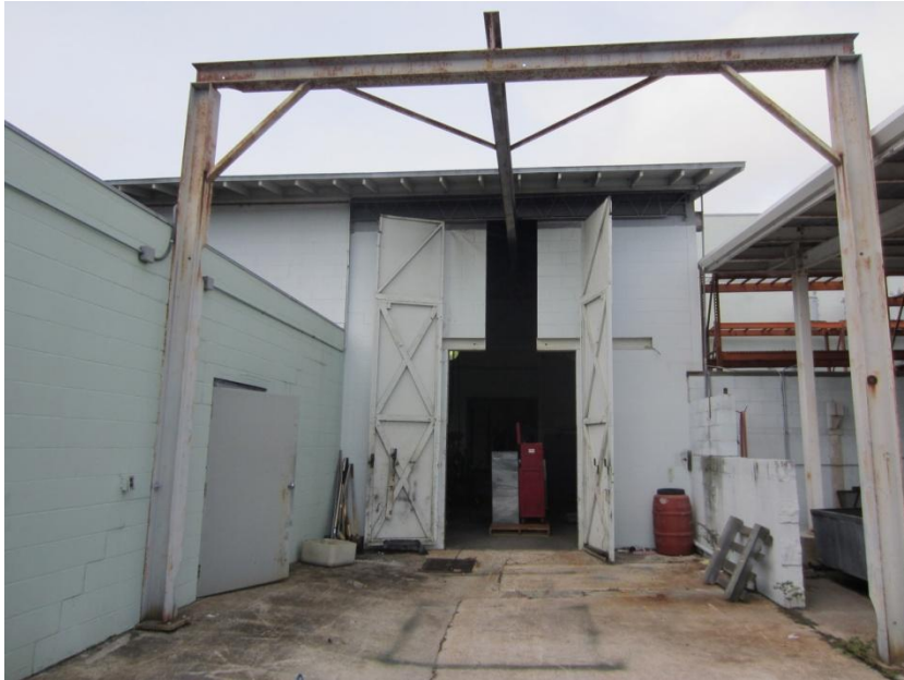
Side Machinery Entry
