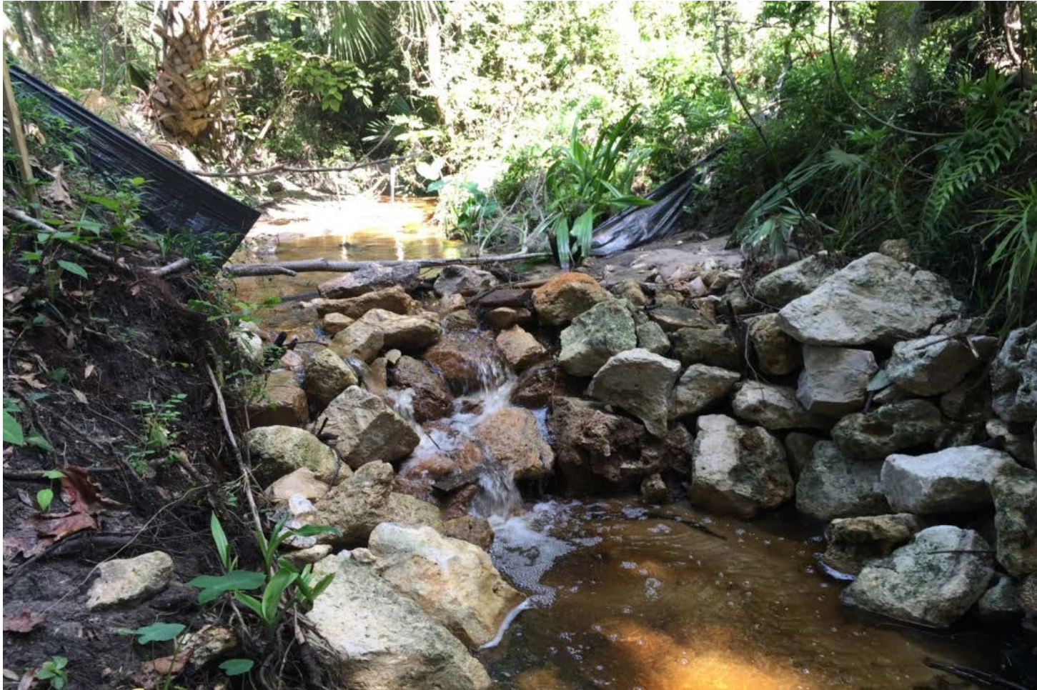
Beville Creek in Cofrin Nature Park during construction (8/19/2015). Large boulders creating a check dam for grade control within Beville Creek.
