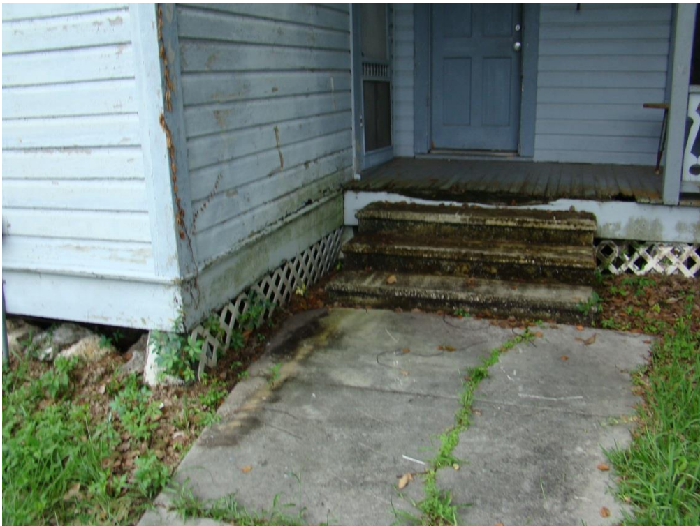
Details of front porch #623.
