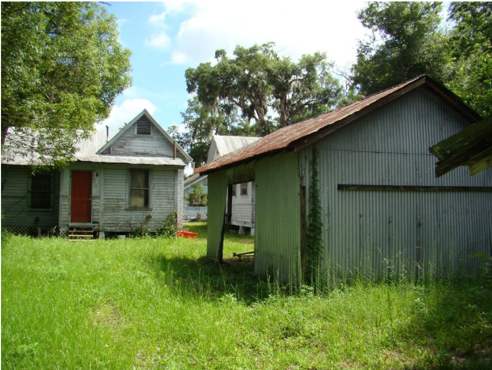
View of non-contributing shed to be demolished.
