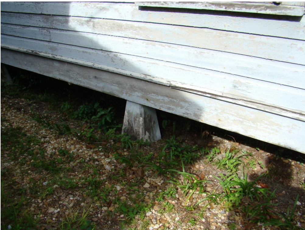
Detail of brackets and roofing #623 (top). Detail of concrete pier (bottom).
