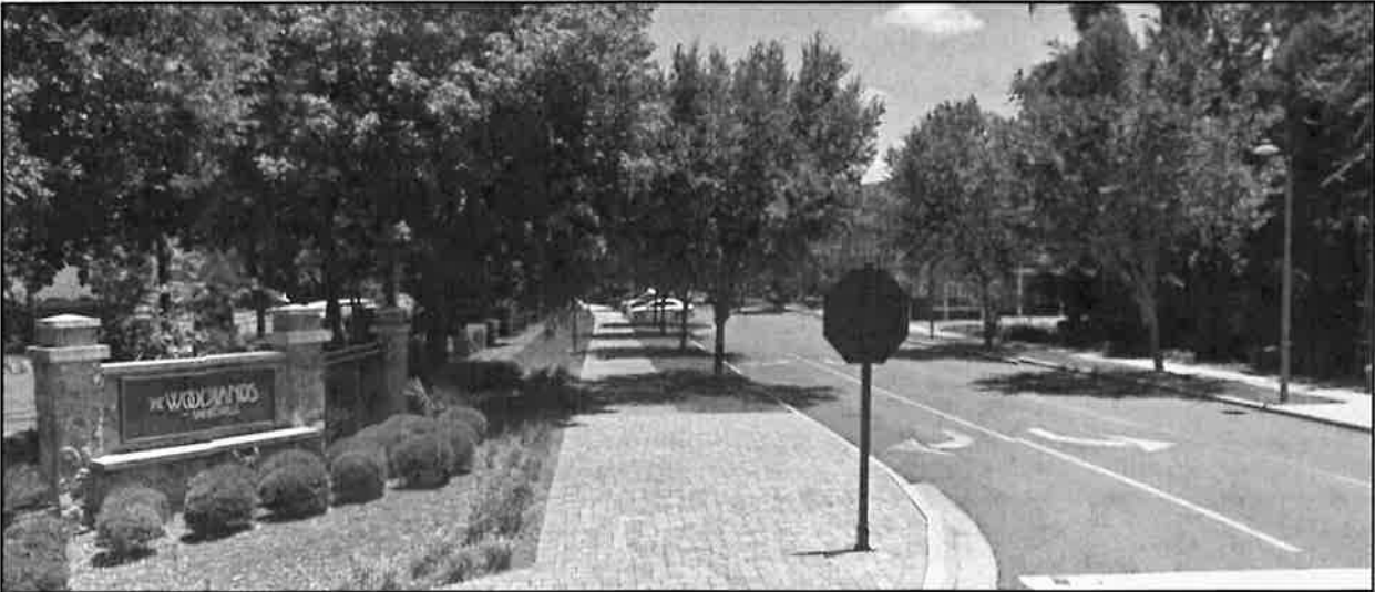
Figure 8: NE Corner of SW 52 nd Street and SW 20 th Avenue Intersection — The Woodlands Apartment Complex
