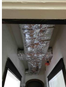
Downstairs AC ductwork
