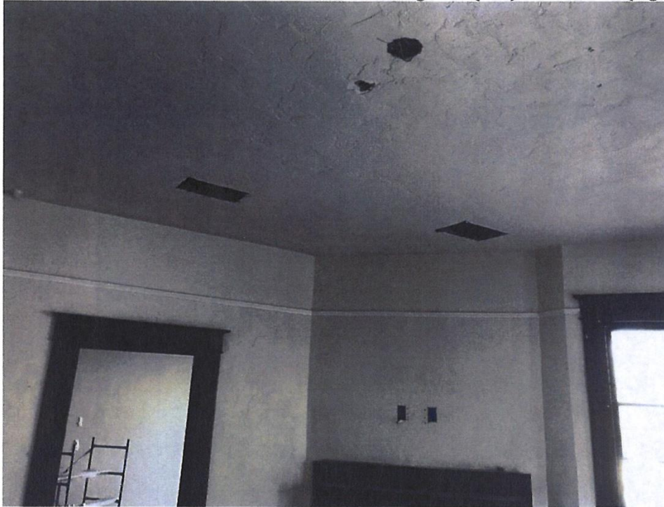
Second floor bedroom 1 – Cut-outs for new register (left) and return (right)
