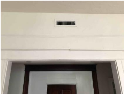
New AC vent in dining room
