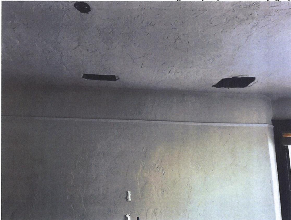
Second floor bedroom 2 – Cut-outs for new register (left) and return (right)
