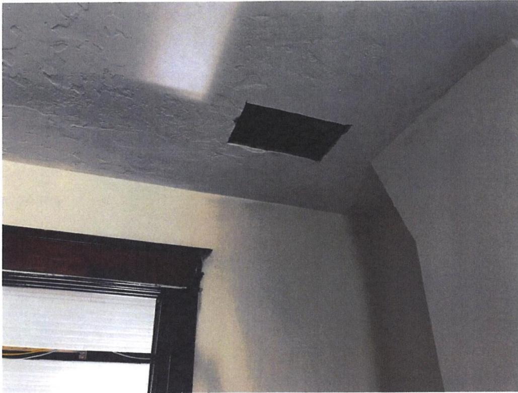
Second floor bedroom - Cut-out indicates return
