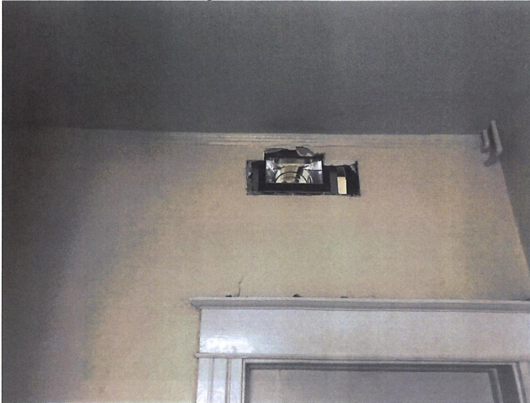
First floor bathroom – New register location over door
