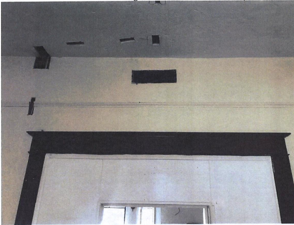
Parlor – Cut-out indicates new register location over doorway
