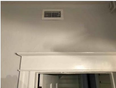
New AC vent in downstairs bath
