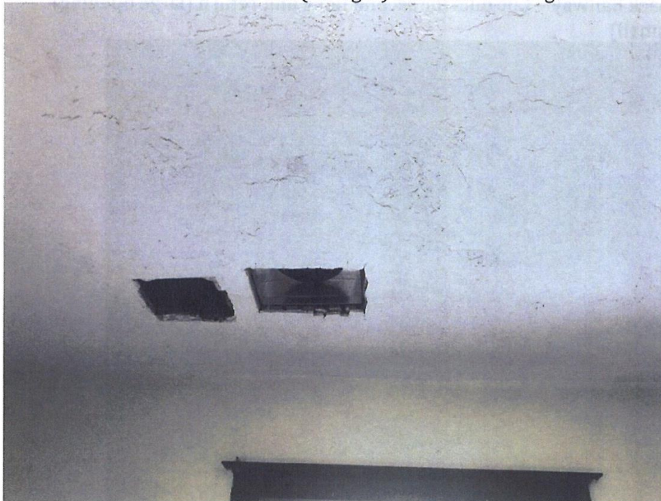
Second floor bedroom – Cut-out (on right) indicates new register location
