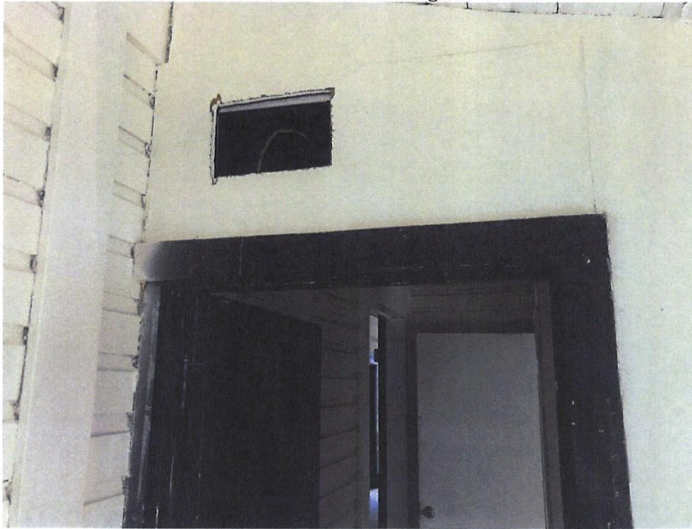
Second floor bedroom – Cut-out (on right) indicates new register location
