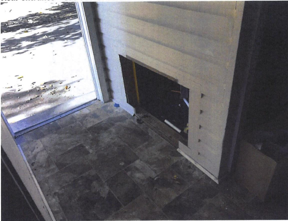
Second floor front hallway - Cut-outs indicate locations for two new registers
