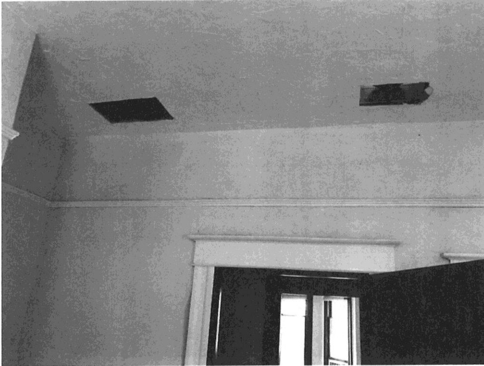
Second floor bedroom 3 – Cutouts for new register (right) and return (left)
