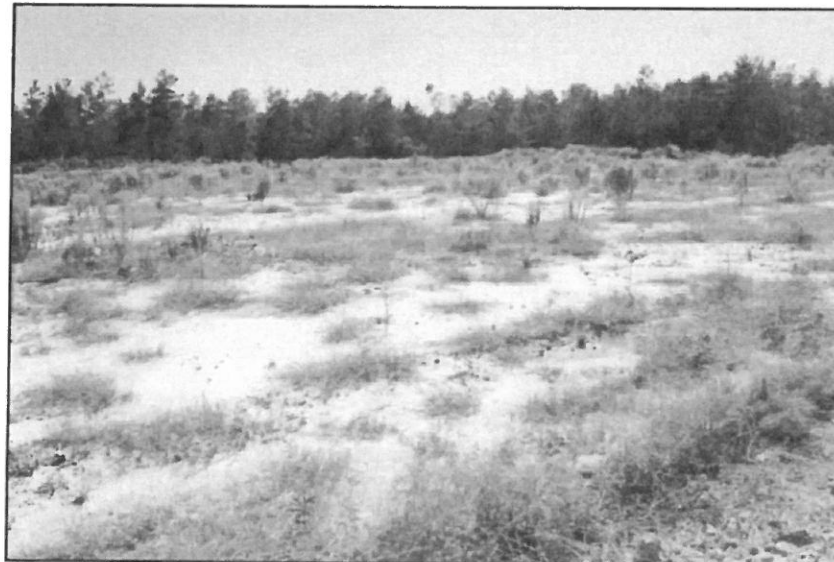
Pilot Study Area - Cleared & Grubbed
